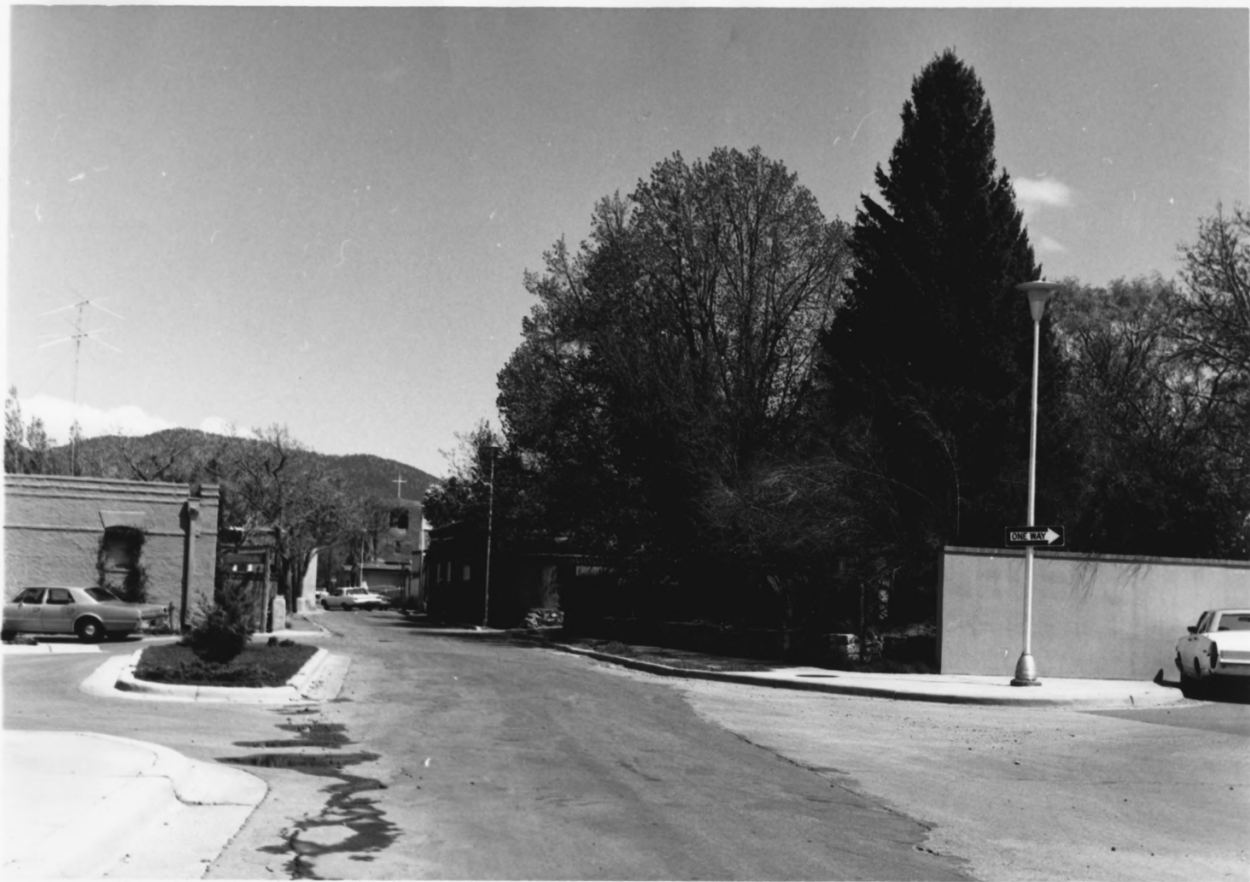
East De Vargas Street, looking east toward San Miguel Church.
