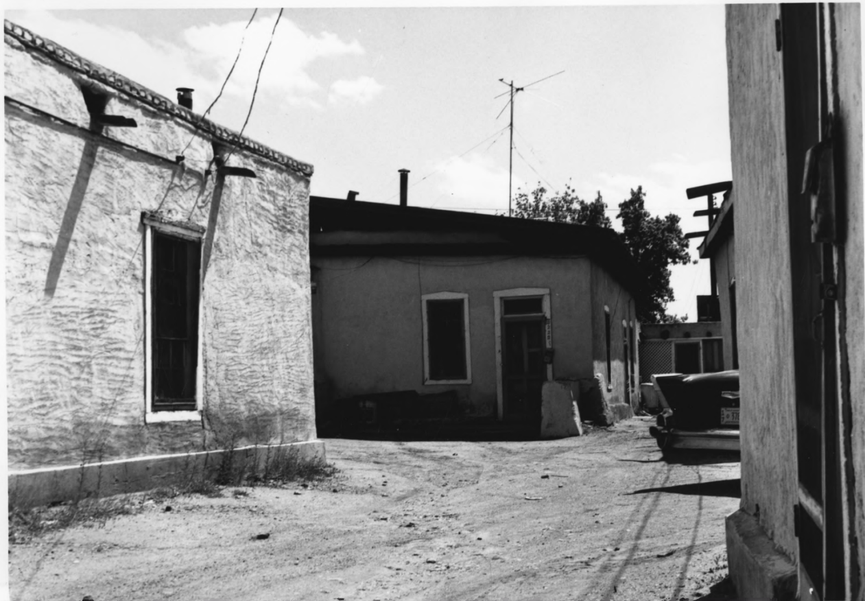
Example of unplanned court arrangement behind West De Vargas Street Facade.
