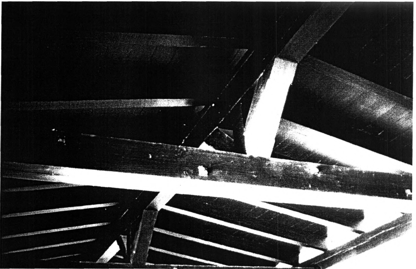
FIGURE 11: Traverse ridge beam detail similar to that of 1947 Chapel. Photo courtesy of the Joesler/Murphey Collection, Arizona Architectural Archives, University of Arizona.
