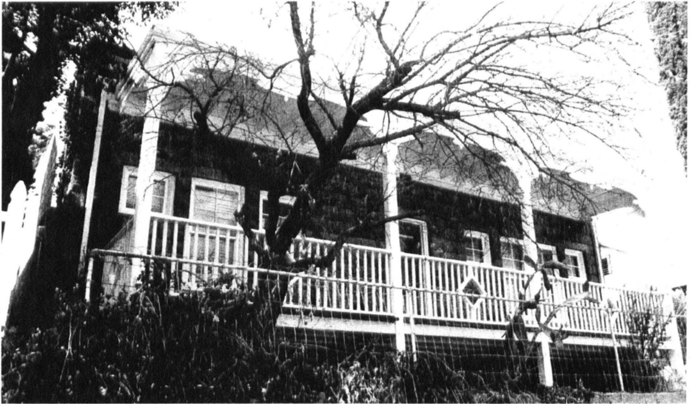
Early concrete block were often formed to resemble roughly cut stone, as in this house at 17 Clawson Avenue (Br-662). Old Bisbee Historic Residential Survey (2002).
