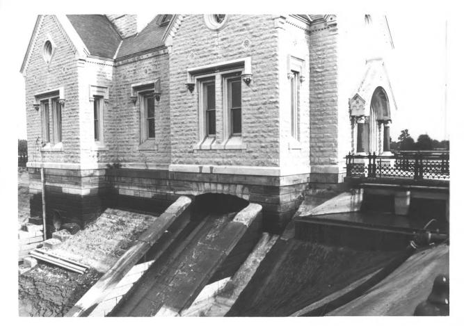
Photo No. 5. Gatehouse looking southeast showing arched sluice opening in foundation.
