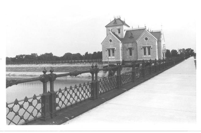
Photo No. 3. Gatehouse looking southeast from promenade. Note cast-iron railing at settling basin perimeter.
