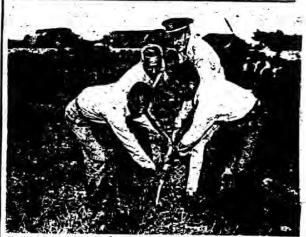
WITH A HEAVE-HO —Governor Pownall and Guam Congress dignitaries dig deep into Agana soil, breaking the ground for the new Guam Congress building. (L to R) Mr. Simson Sanchez, secretary of the house of council; Mr. E. J. Bordallo, chairman of the house of council; Admiral Pownall and Mr. Frank Perez, secretary of the house of assembly. (Navy News Photo)
