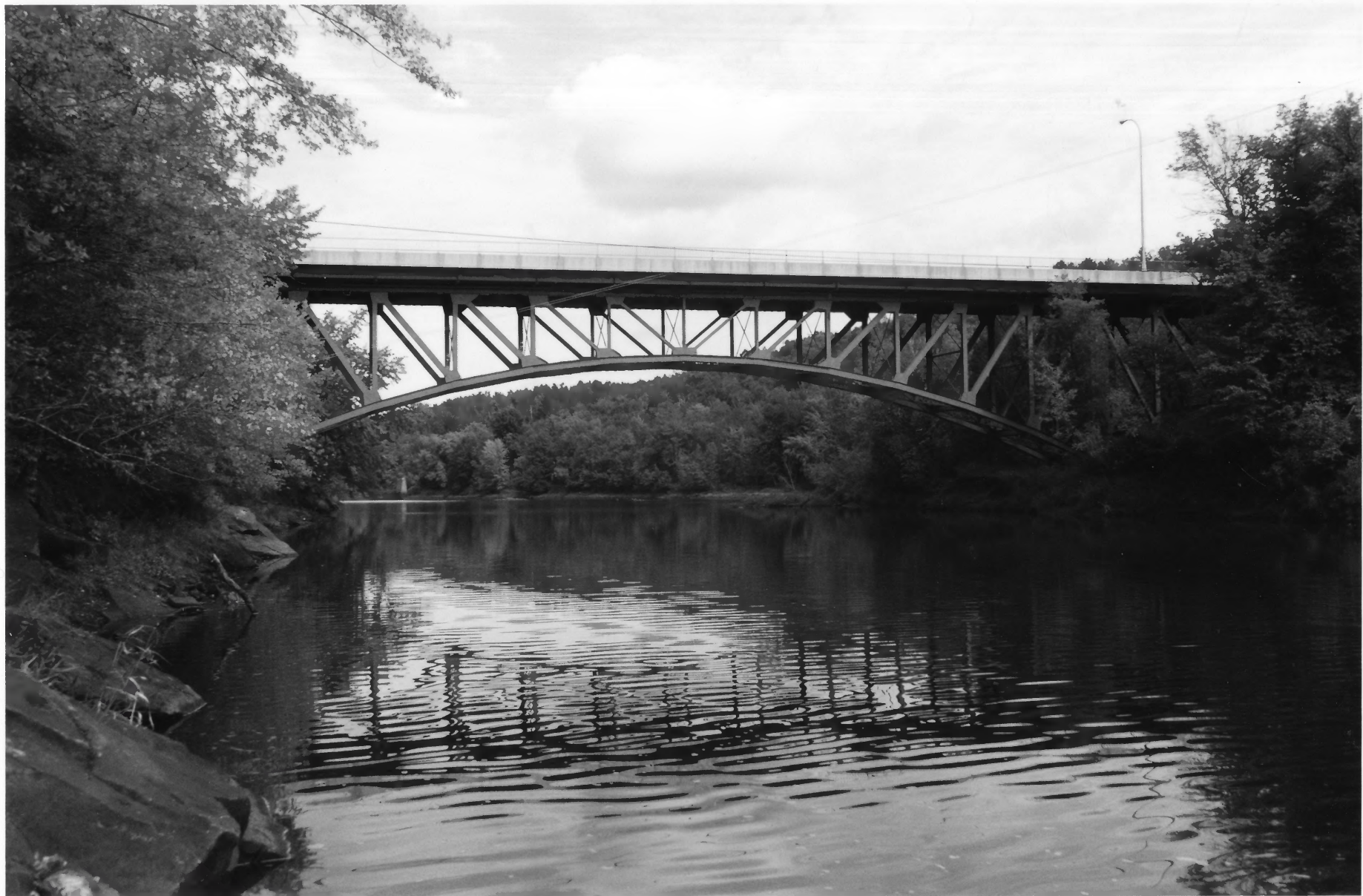
Kettle River Bridge (Bridge no. 5718) Mn Highway 123 over Kettle River, Sandstone Pine Co., Mn 013085/11
