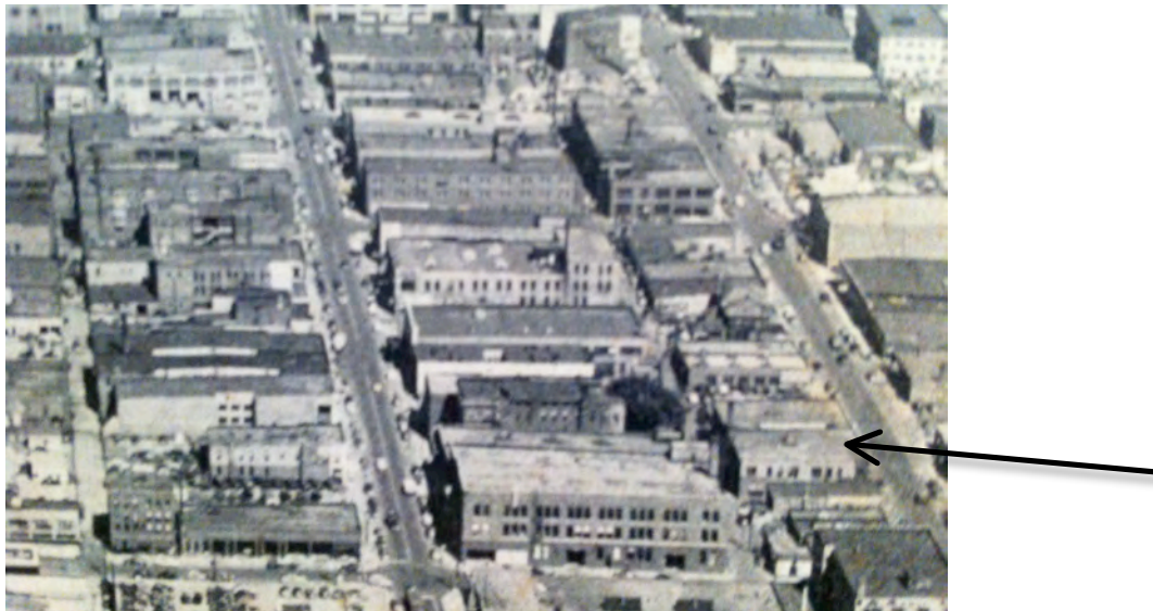
Image 10: This detail of a circa-1951 aerial photo of the “West End” Auto Row district, taken looking east, shows Locust Street (left) and Walnut Street (right). The arrow points to 1417-1425 Walnut Street. (The American Swedish Monthly, July 1951)
