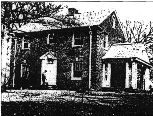
Figure 94: 515 Foster Drive, Completion photo ( Tribune , April 27, 1932)
