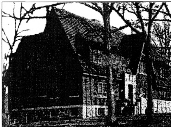
Figure 98: 669 Foster Drive: Construction completion photo ( Register , December 1, 1929).
