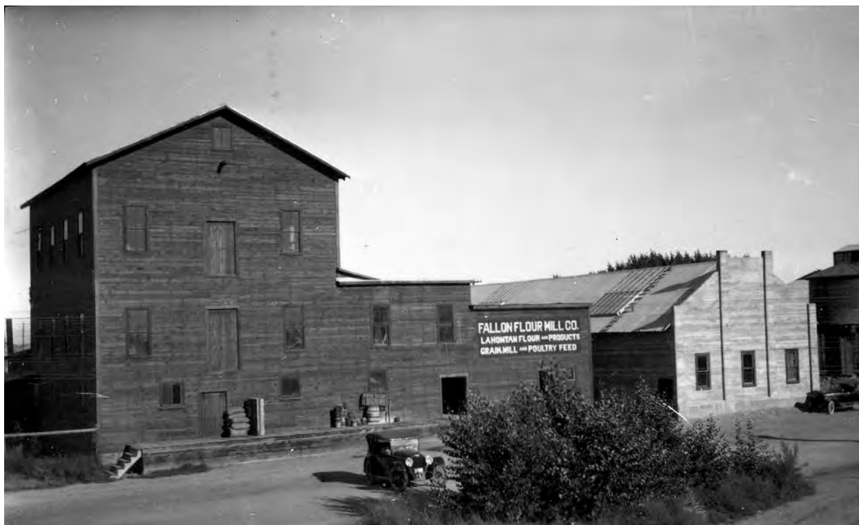
Figure 4: The Fallon Flour Mill on North Maine Street, c.1925, showing the frame mill building prior to its burning and demolition. The warehouse at the right of the photo remains (Special Collections, University of Nevada, Reno).
