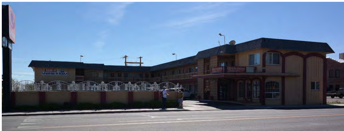
Photographs 21: (Right) Econo Lodge at 70 East Williams, looking south (Campana, 2015).
