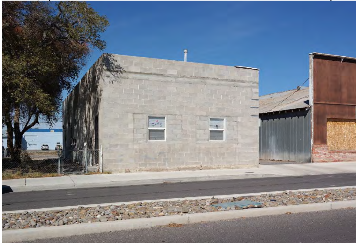
Photograph 13: The Clayton Building at 135 East Center Street, looking north off Center Street (Campana, 2015).
