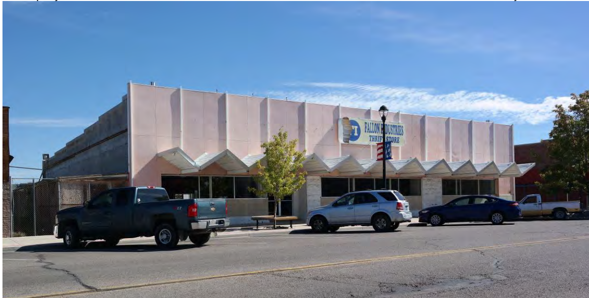
Photograph 63: 165 South Main Street, the I.H. Kent Company's main store, with a post-1954 Mid-Century Modern slip cover, among the best examples of mid-century architecture in Fallon (Campana, 2015).
