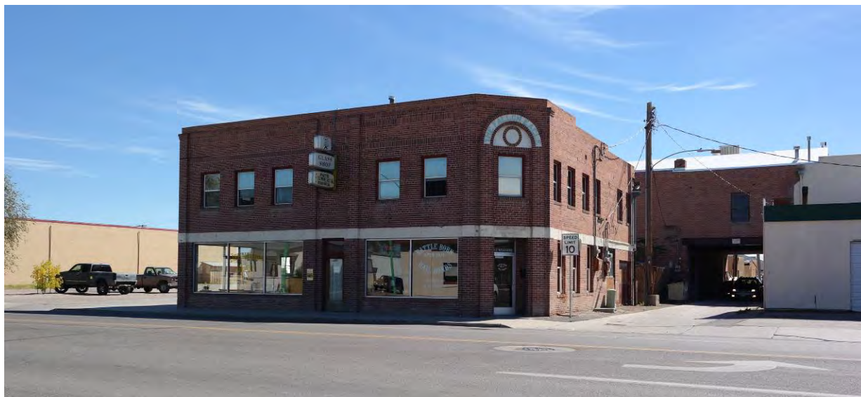
Photograph 18: The Fallon Eagle Building at 42 East Williams, looking southeast (Campana, 2015).
