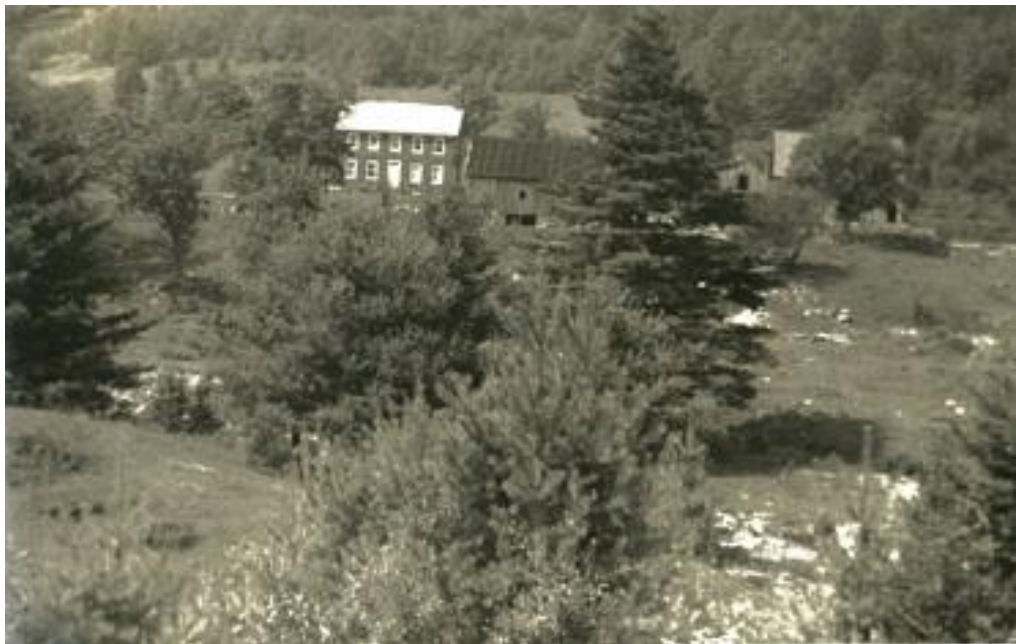
Facing southwest toward house, former outbuildings, and extant barn, c. 1940s
