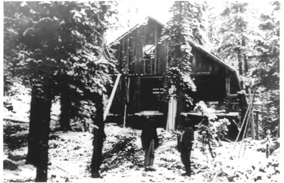
Photo 2: Maycock cabin under construction (circa 1927)
