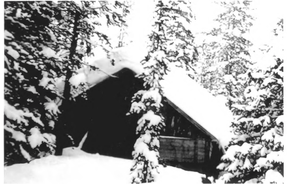
Photo 4: Maycock cabin under construction (circa 1927)
