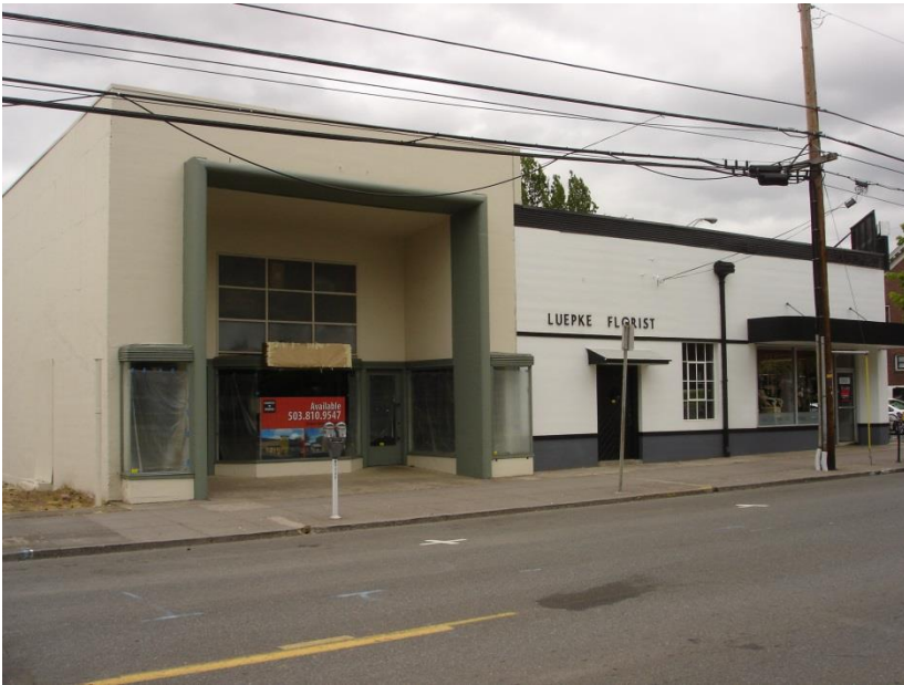
Name of Property: Luepke Florist City or Vicinity: Vancouver County: Clark State: Washington Photographer: Holly Chamberlain Date Photographed: 11 July 2015 Description of Photograph(s) and number: south elevation
