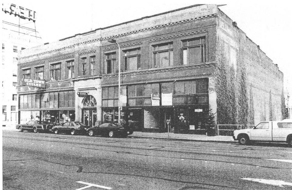
PHOTO No. 17—AUGUST 1998 PHOTOGRAPH OF THE DAYLIGHT BUILDING'S SOUTHEAST FRONT FACADE. SOURCE: WHATCOM MUSEUM OF HISTORY AND ART, GORDON TWEIT COLLECTION, 1998.77.62.
