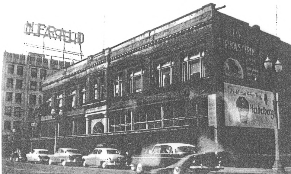
PHOTO No. 15—Ca 1950s PHOTOGRAPH OF THE DAYLIGHT BUILDING'S FRONT FACADE. SOURCE: WHATCOM COUNTY ASSESSOR'S OFFICE.
