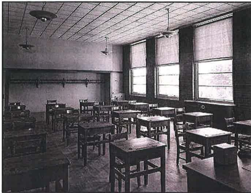
Figure 3 – typical classroom (c. 1942)
