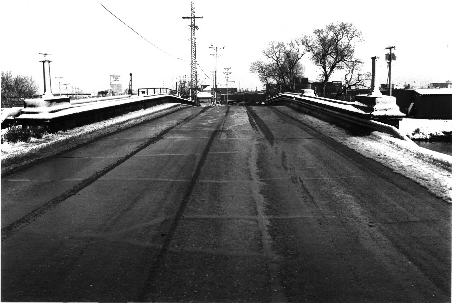
NUMORE BRIDGE # 2366 BELTRAMI CO., MN PHOTO I.D. 09352 #8
