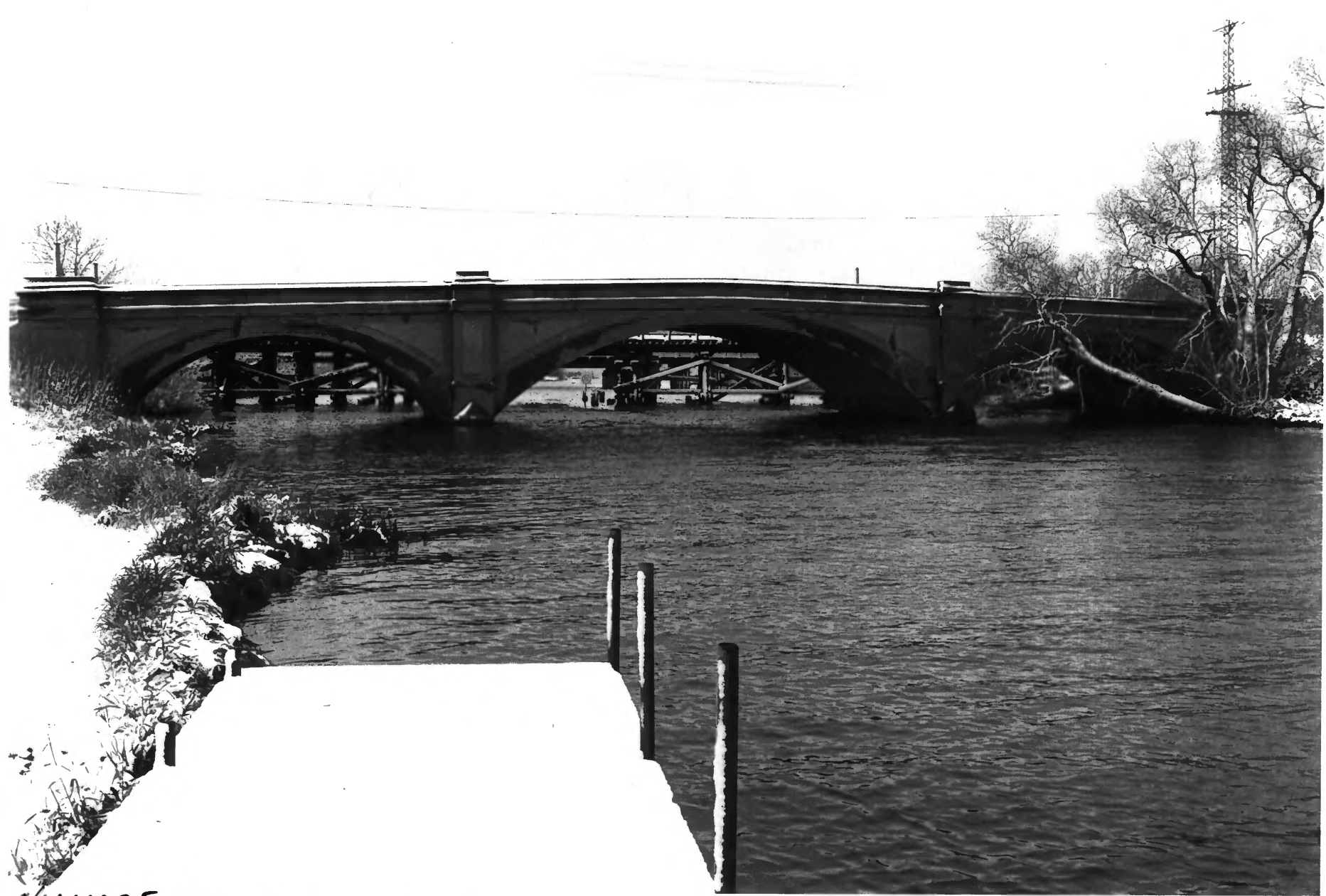
NUMORE BRIDGE # 2366 BELTRAMI CO., MN PHOTO I.D. 09352 #10
