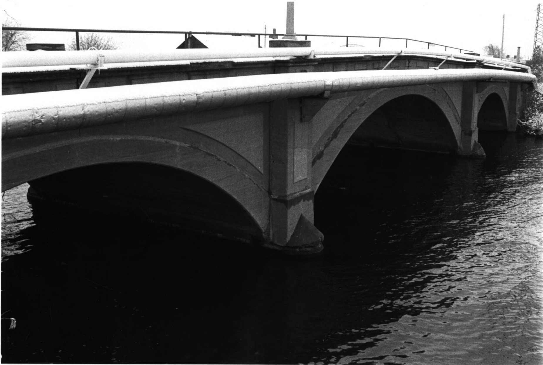
NYMORE BRIDGE #2366 BELTRAMI CO., MN PHOTO I.D. 09352#15
