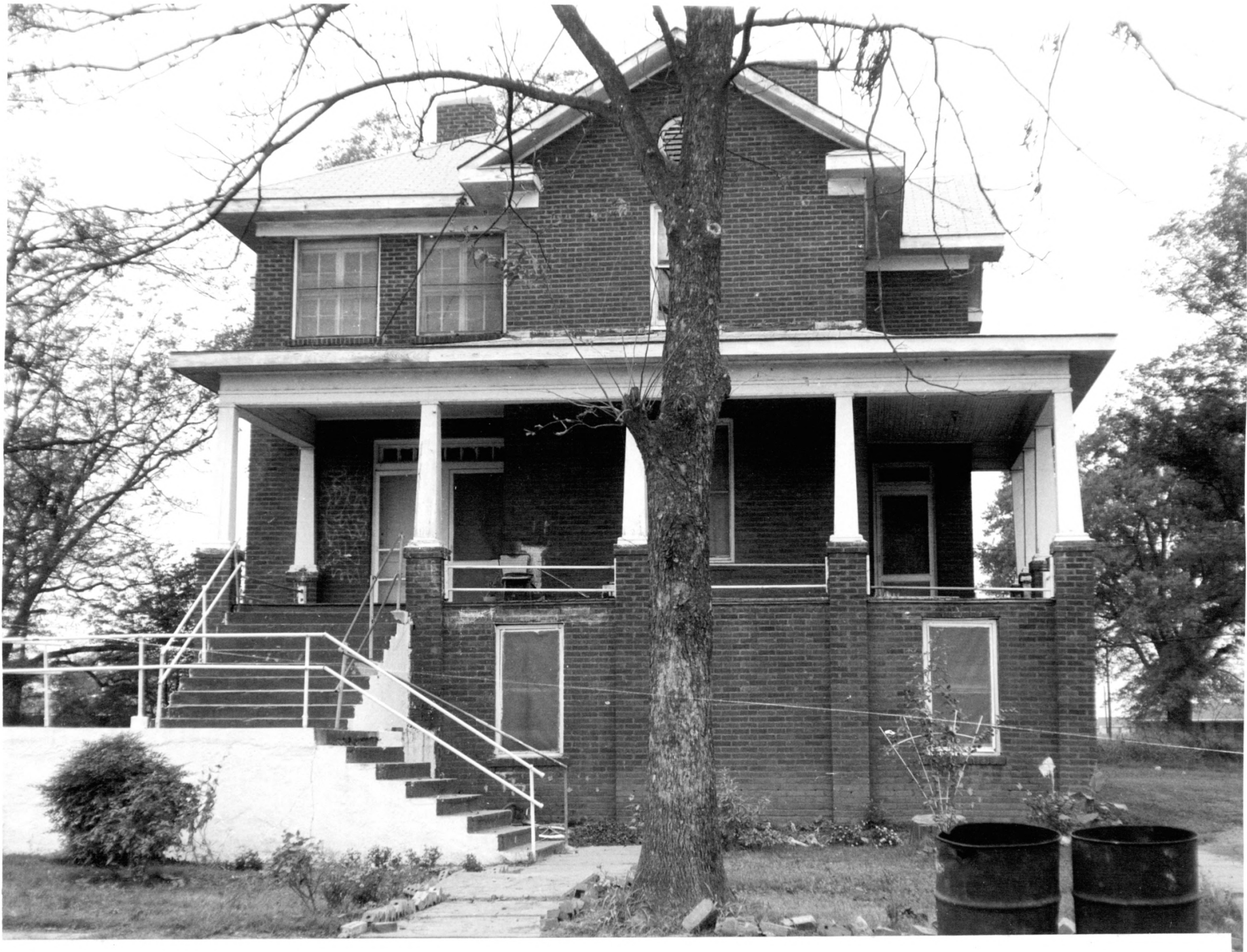
I. T. Montgomery House, Mound Bayou, Mississippi East facade looking west
