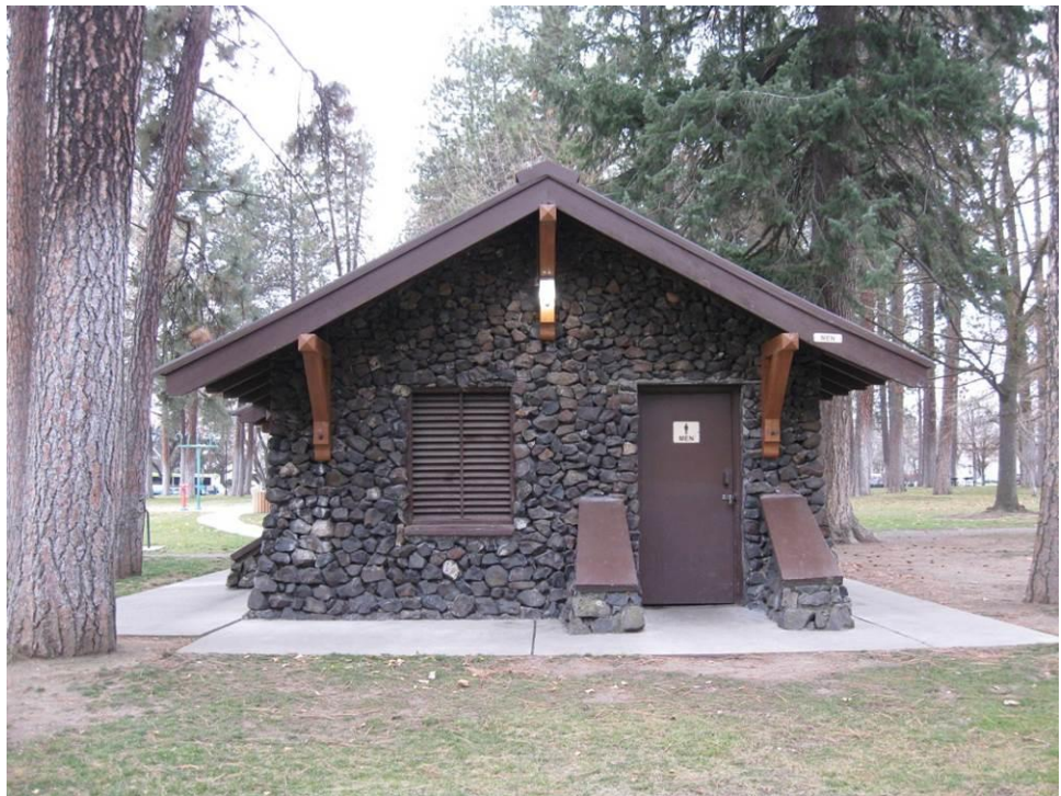
Photo 15. WA_SpokaneCounty_CoeurDALenePark_0015. Restroom, Men's side, view west.
