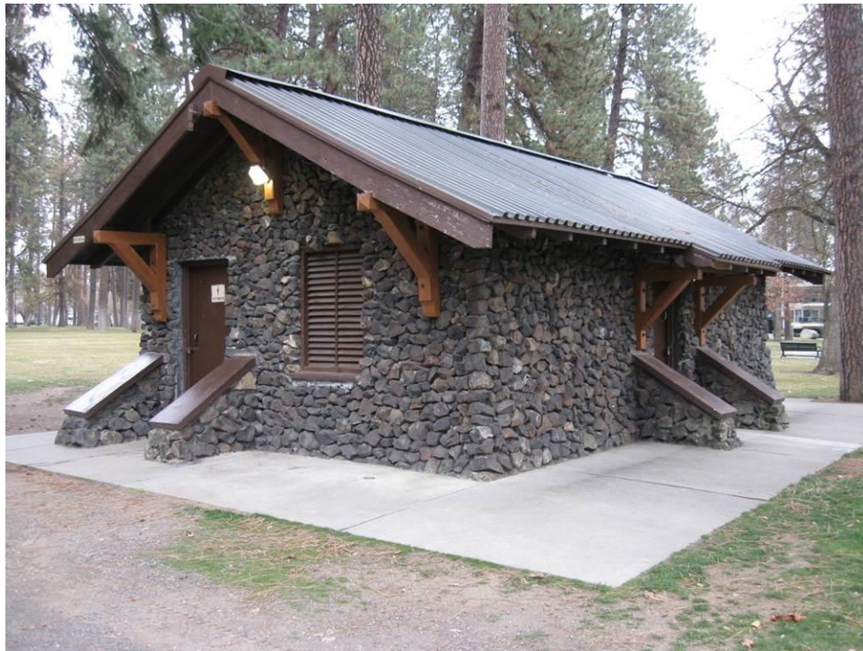
Photo 17. WA_SpokaneCounty_CoeurDALenePark_0017. Restroom, oblique, view northeast.
