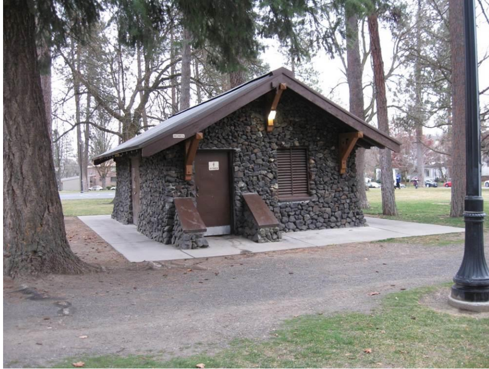
Photo 16. WA_SpokaneCounty_CoeurDALenePark_0016. Restroom, Women's side, view southeast.
