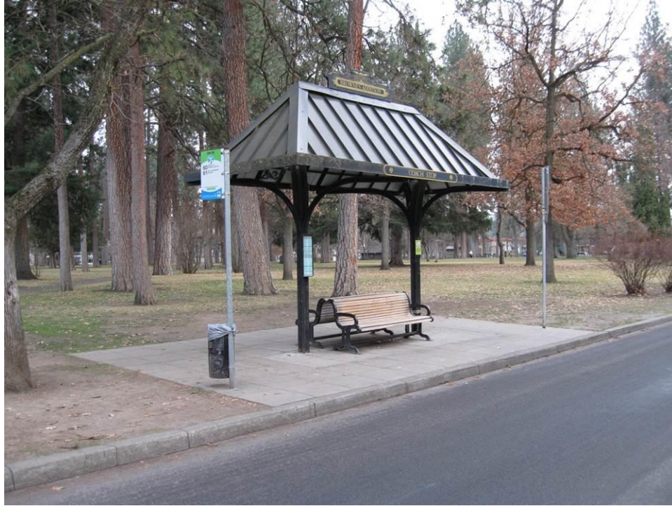
Photo 10. WA_SpokaneCounty_CoeurDALenePark_0010. Bus Stop Shelter, view southeast.
