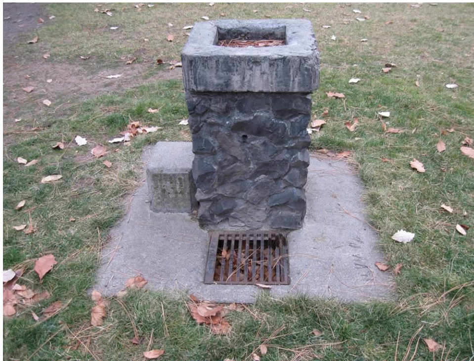
Photo 13. WA_SpokaneCounty_CoeurDALenePark_0013. Stone Drinking Fountain with drain, view east.
