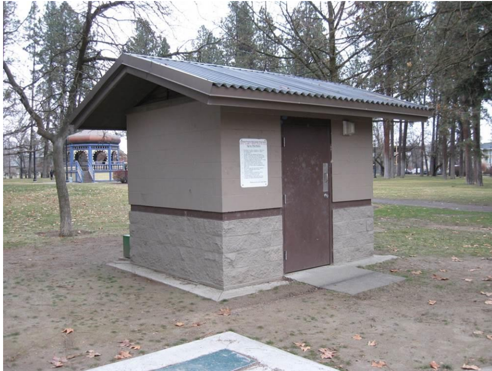
Photo 8. WA_SpokaneCounty_CoeurDALenePark_0008. Maintenance/Controls Shed, view northeast.
