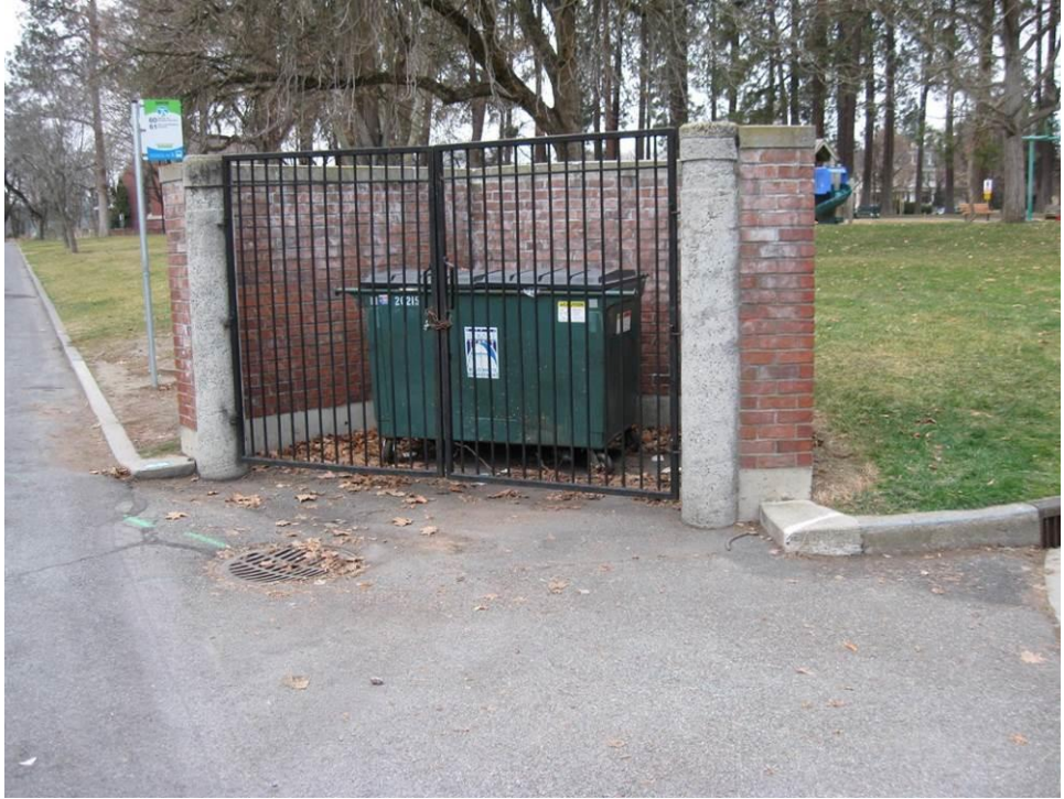
Photo 4. WA_SpokaneCounty_CoeurDAlenePark_0004. Brick Dumpster Enclosure, view northwest.
