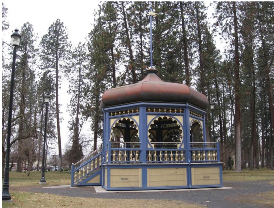
Photo 19. WA_SpokaneCounty_CoeurDALenePark_0019. Pavilion, view west.
