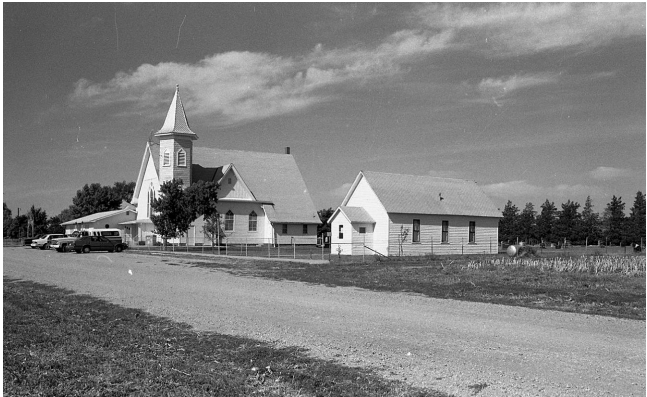
Figure 8: Immanuel Lutheran Church, also known as State Line Church, in 1991. The complex preserves its original organization including school, church, parsonage, and cemetery. A large addition to the front of the wood-frame church (visible on the left) reduces its integrity somewhat. (GA00-019, Gage County Survey Image, 1991)
