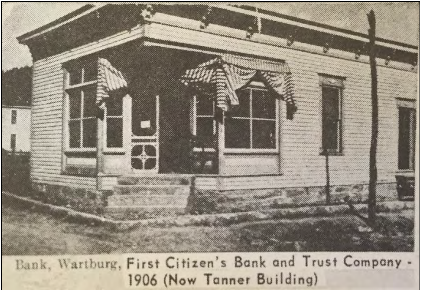
Figure 3: 1910 photograph of c.1906 Citizens Bank and Trust section. From a 1910 postcard photographed by Bruno Schubert. Source: Morgan County News , 1981.
