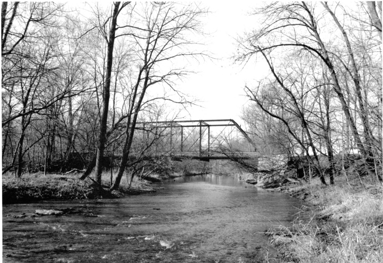
#1 Rush County Bridge #188
