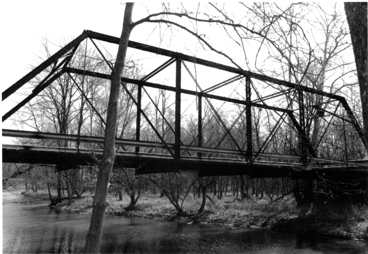
#2 Rush County Bridge #188
