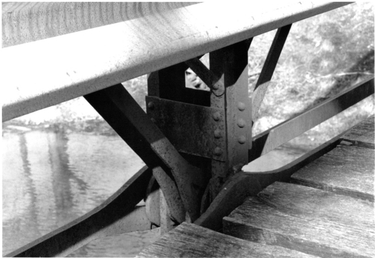
#7 Rush County Bridge #188
