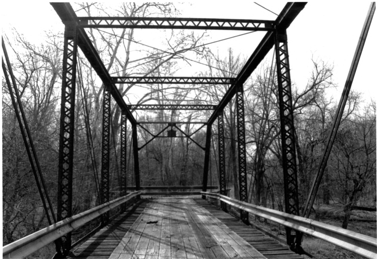
#5 Rush County Bridge #188
