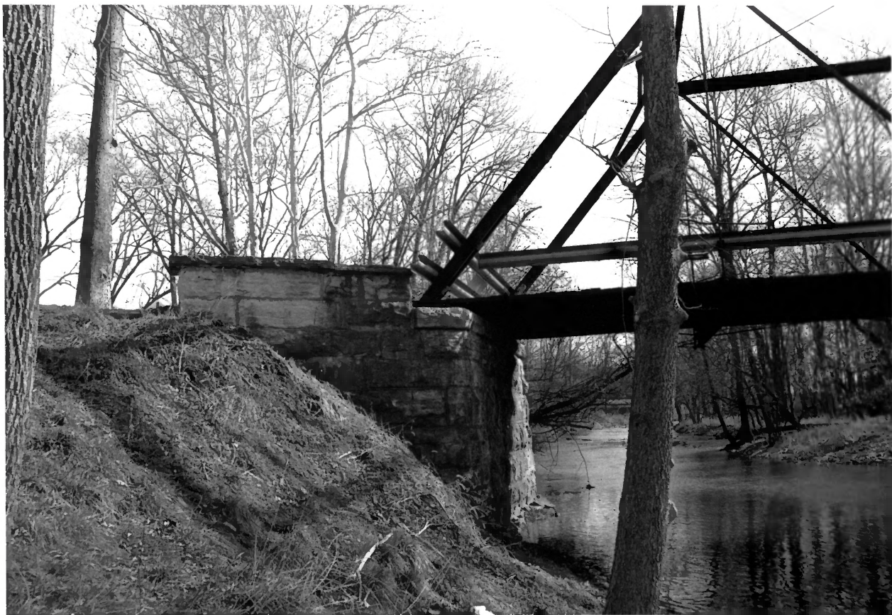
#3 Rush County Bridge #188
