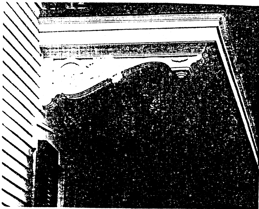
See classic wooden frame's ornamental brackets in detail in this close up in front gallery
