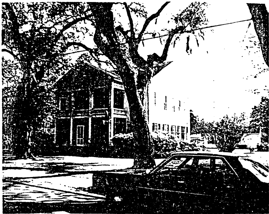
Three-quarter view shows symmetrical window arrangements. Note outbuildings at rear.
