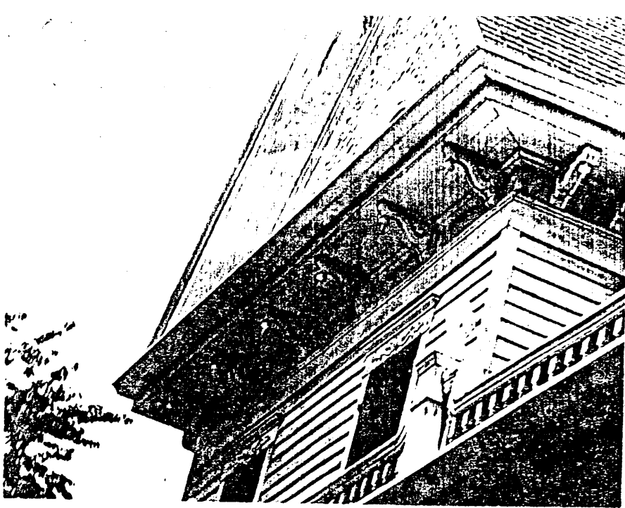
Window brackets, brackets, hood, pediment show up in this detail shot of the front gallery
