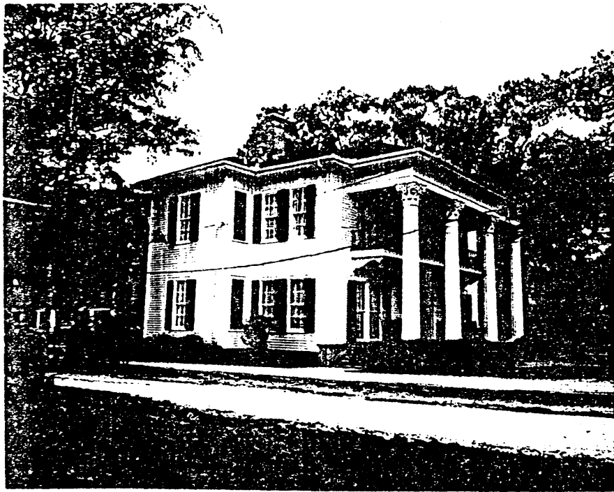
Three quarter view shows side elevation, and additions at rear.
