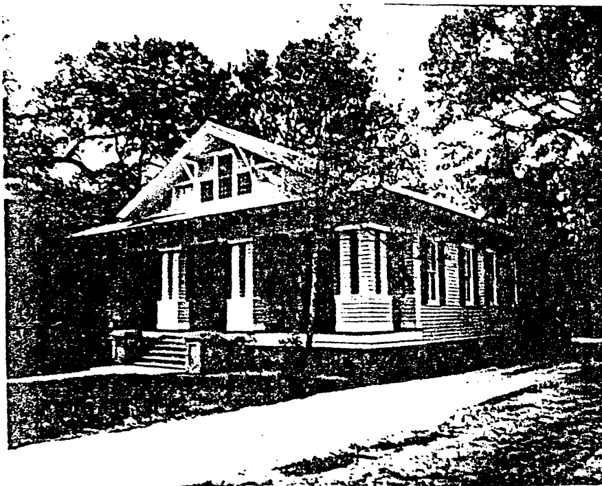
Three quarter view shows matching engaged columns against gallery walls. Note bungalow brackets on roof overhang at front.
