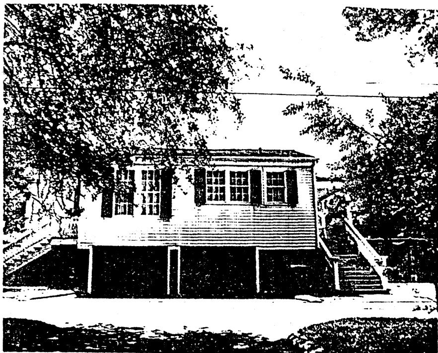
Another view of side entrance and main porch and staircase.
