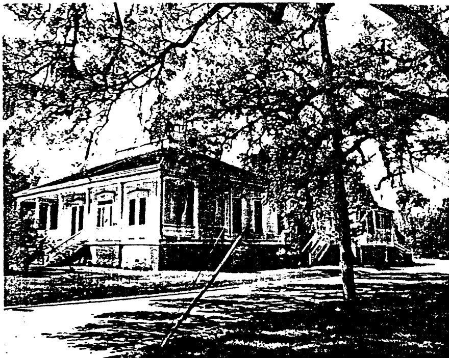
View of opposite side - note addition on rear side
