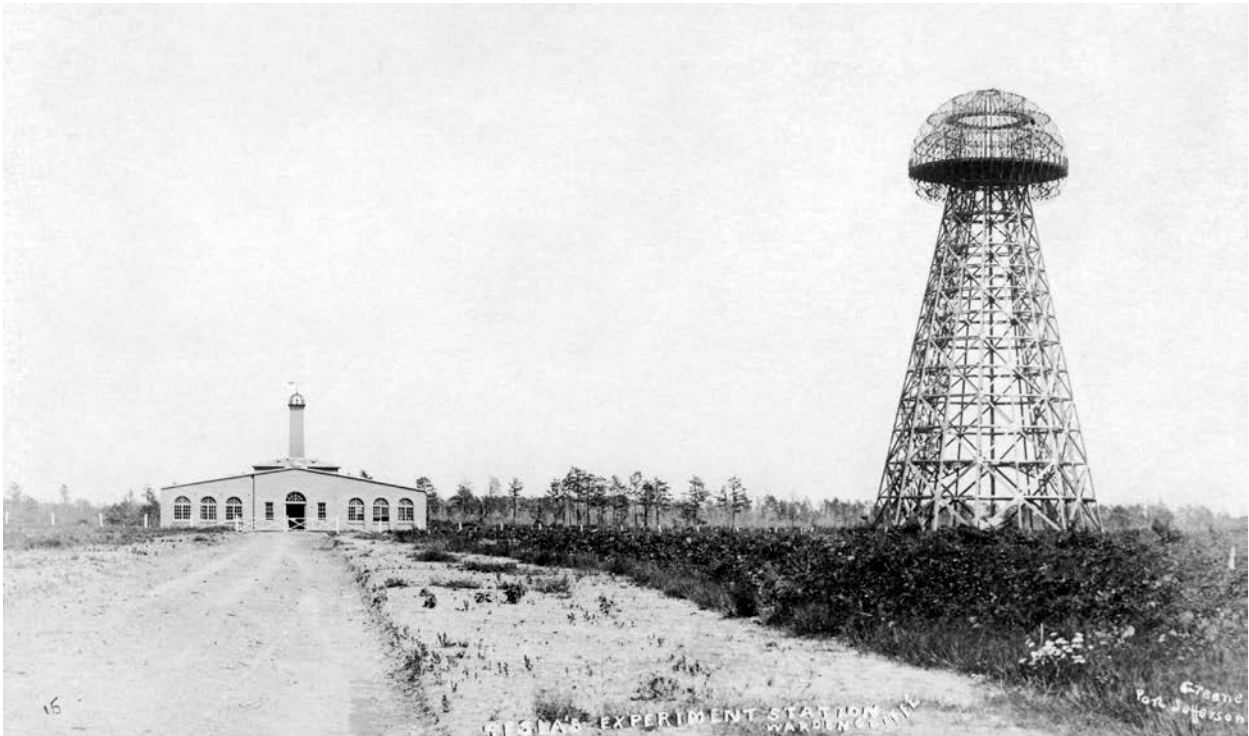
Figure 4. West elevation of Wardencllyffe, approaching from Randall road after tower dome added. Photograph signed Greene, Port Jefferson, circa 1903-1917.
