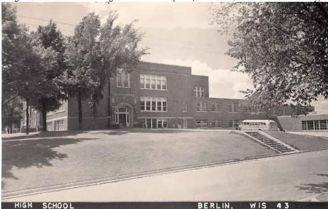
Figure 8: View of east façade, including the 1955 addition (date known; Berlin Historical Society)
