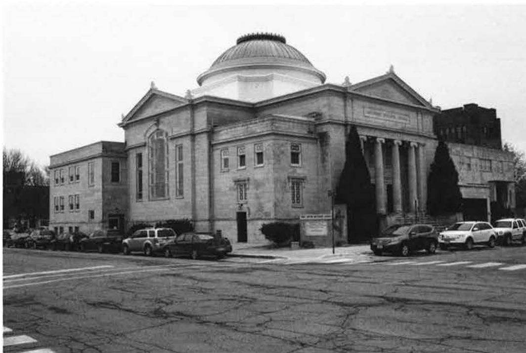
Figure 15. District Photograph: First Methodist Episcopal Church
