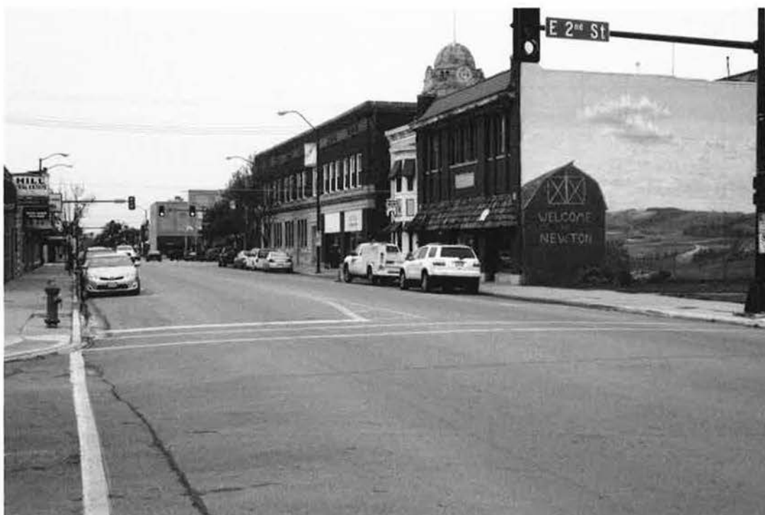
Figure 7. District Photograph: Streetscape with the Joy Dental Building
