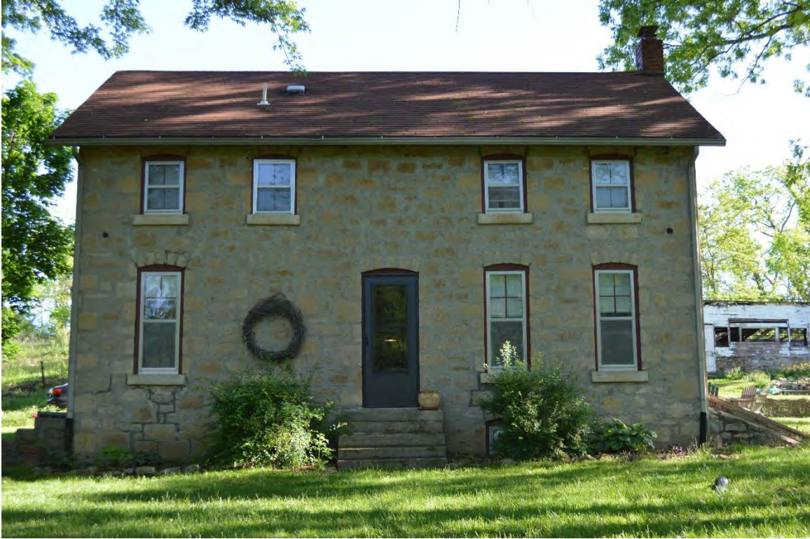
Figure 1. Front (south) elevation viewed to the north, the original entrance to the residence
