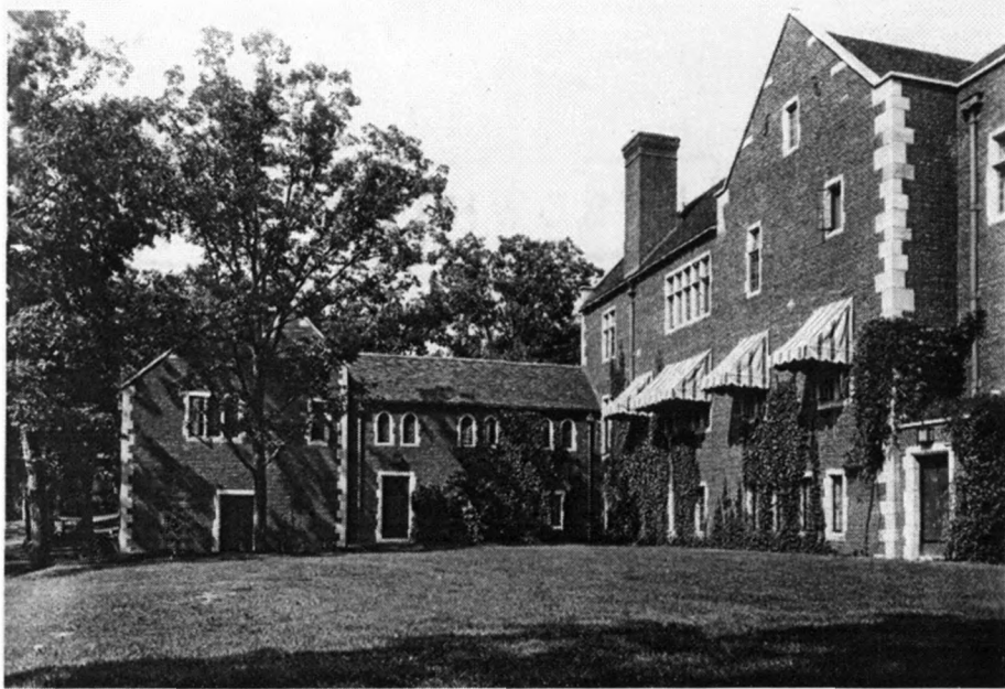
Exterior, west elevation of main house and south elevation of Friendship Hall and garage, looking northeast, c. 1928 (Salisbury House Archives)
