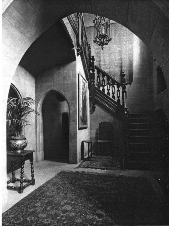
Interior, Main Stair hall, looking east, c. 1928 (Salisbury House Archives)
