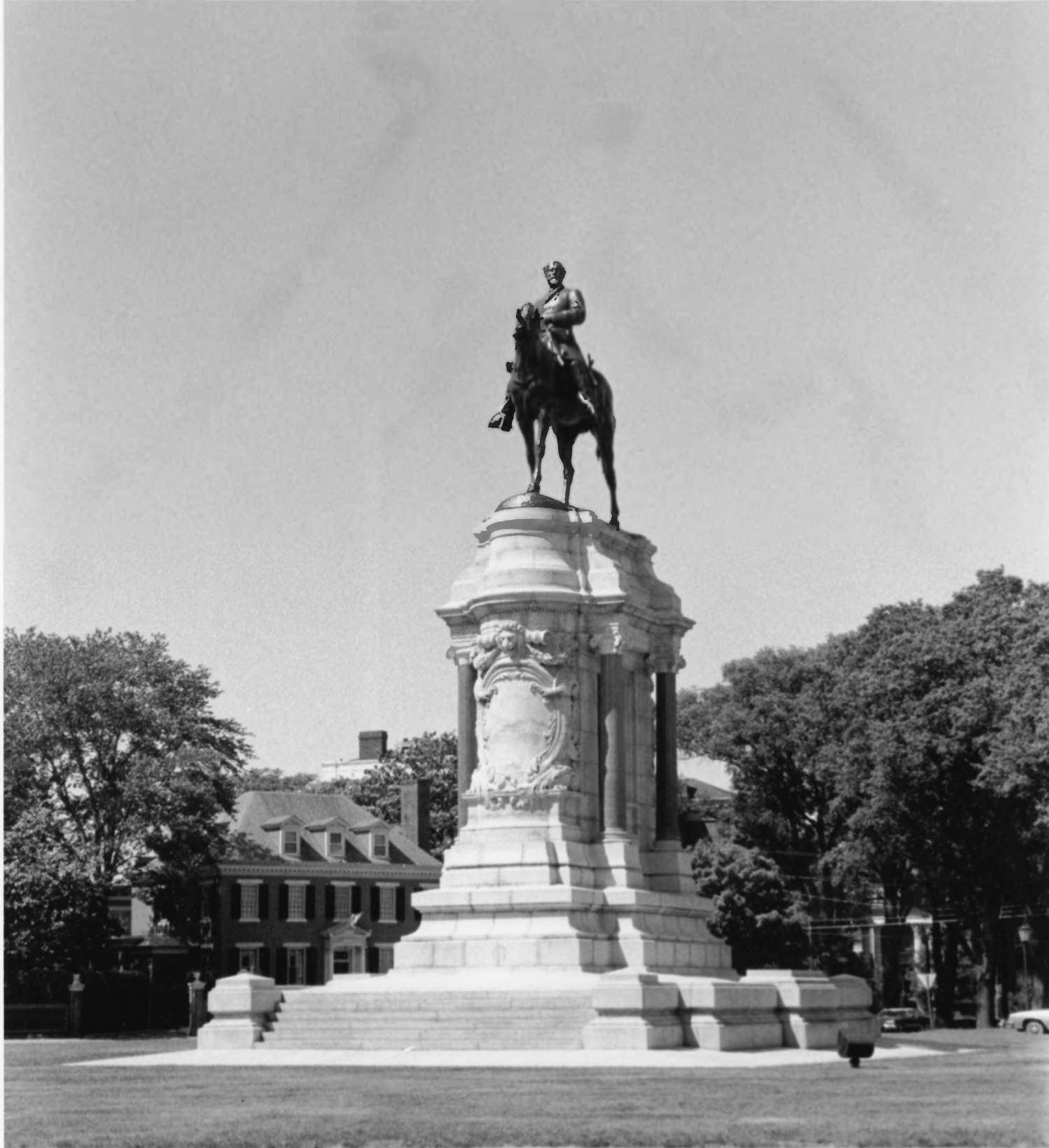
Monument Avenue Historic District Richmond, Virginia Lee Monument & 1800 Monument Ave., The Jeffress House looking northwest Photo: Sarah Driggs, June 1997
