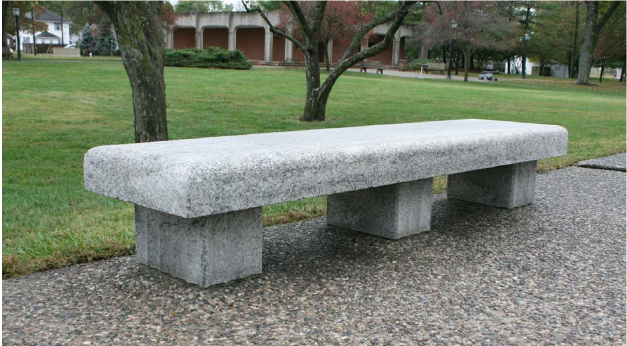
Figure 36. One of the granite benches installed in 1933. The existence of the slightly raised pedestal under the bench supports suggests that the bench may be resting on one of the remaining slabs of original exposed aggregate concrete. Laura L. Knott, October 19, 2011.
