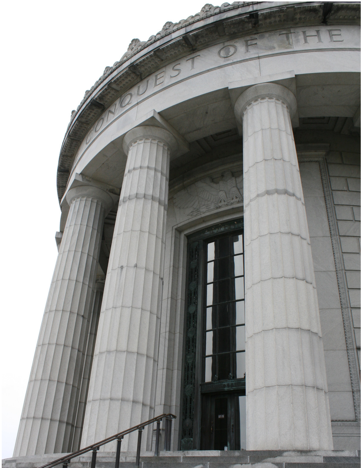
Figure 21. Monumental main entrance on the north side of the Memorial Building. The inscription and detailed cornice are visible at the top. Its fluted columns and cast bronze doors frame the entrance, which is surmounted by a stylized eagle carved in granite. Laura L. Knott, October 19, 2011.
