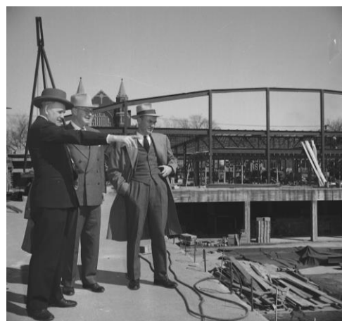
Figure 1: Men observing the construction of the Central Annex, with the building's varying structural systems shown in the background (Courtesy of Sioux City Public Museum).
