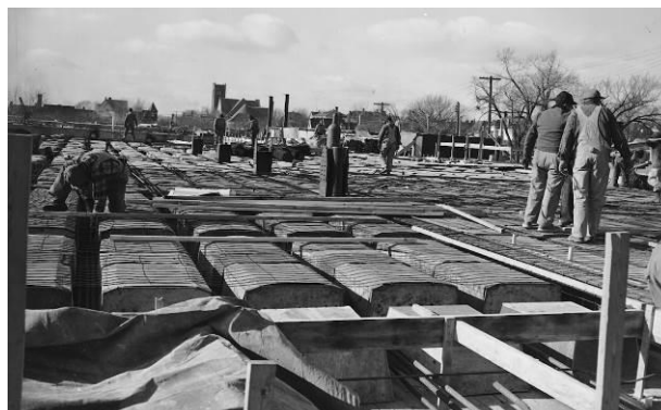
Figure 2: The Central Annex under construction (Courtesy of Sioux City Public Museum)
