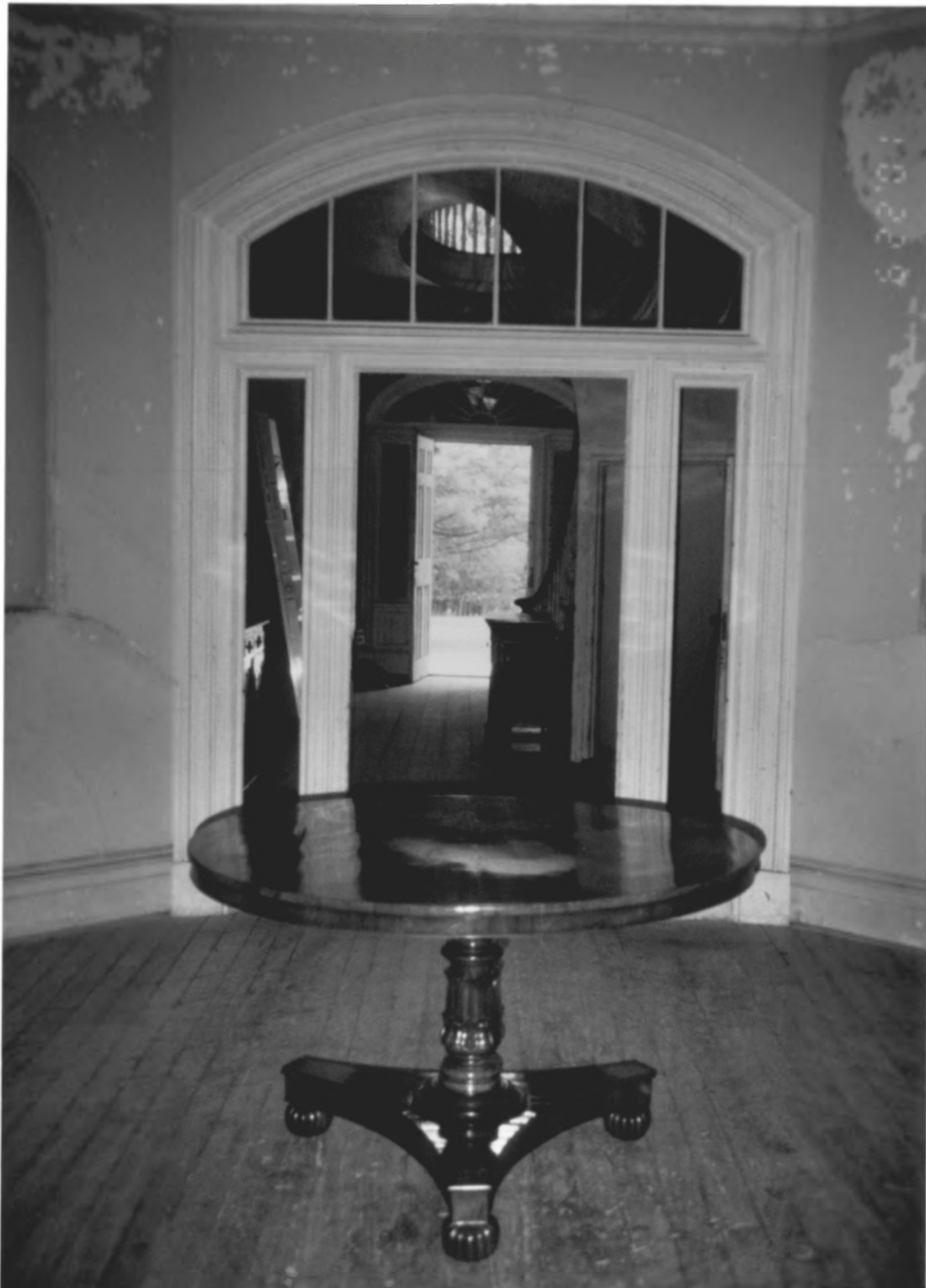
DR. OLIVER BRONSON HOUSE AND ESTATE Hudson, New York View from octagonal hall, first-story, toward east stair hall and vestibule Photo by Peter Shaver and Bill Krattinger, 2001
