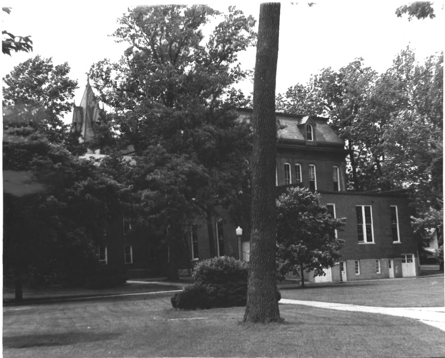
(4) East side of building
