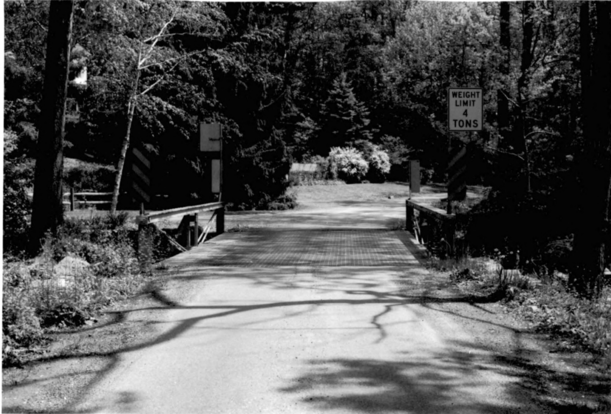
HOLLOW BROOK ROAD BRIDGE, TEWKSBURY TWP., HUNTERDON CO. PHOTO 1 OF 5
