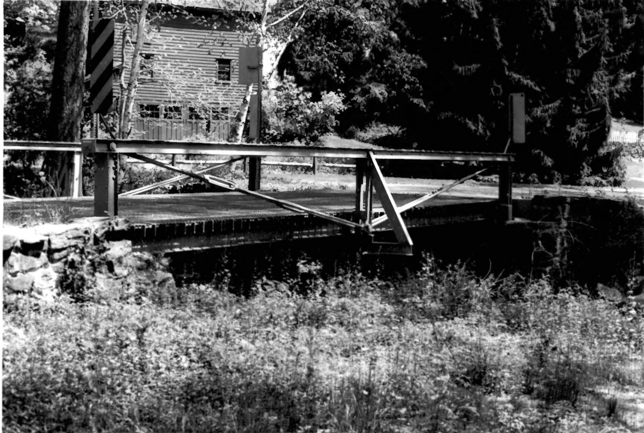
HOLLOW BROOK ROAD BRIDGE, TEWKSBURY TWP, HUNTERDON CO. PHOTO 3 of 5
