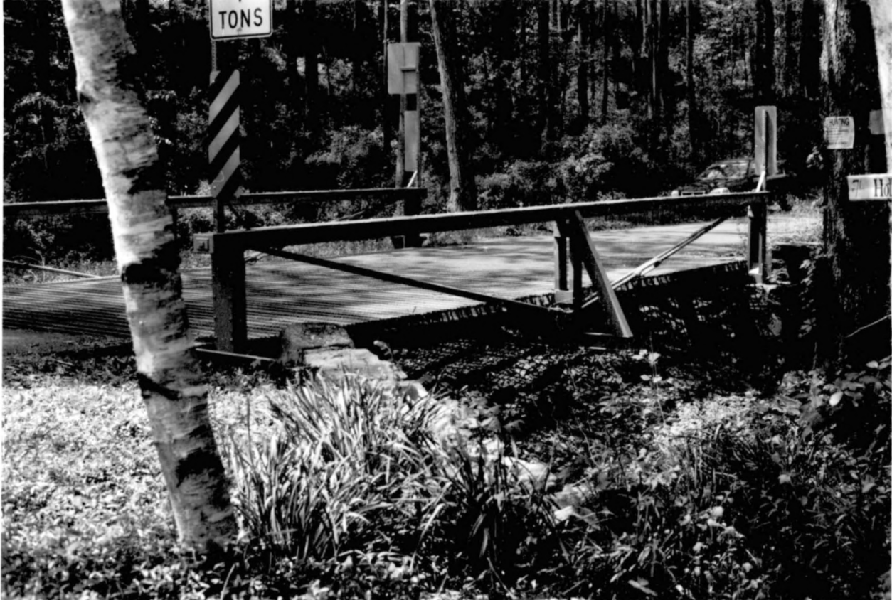
HOLLOW BROOK ROAD BRIDGE, TEWKSBURY TWP., HUNTERDON CO. Photo 4 of 5
