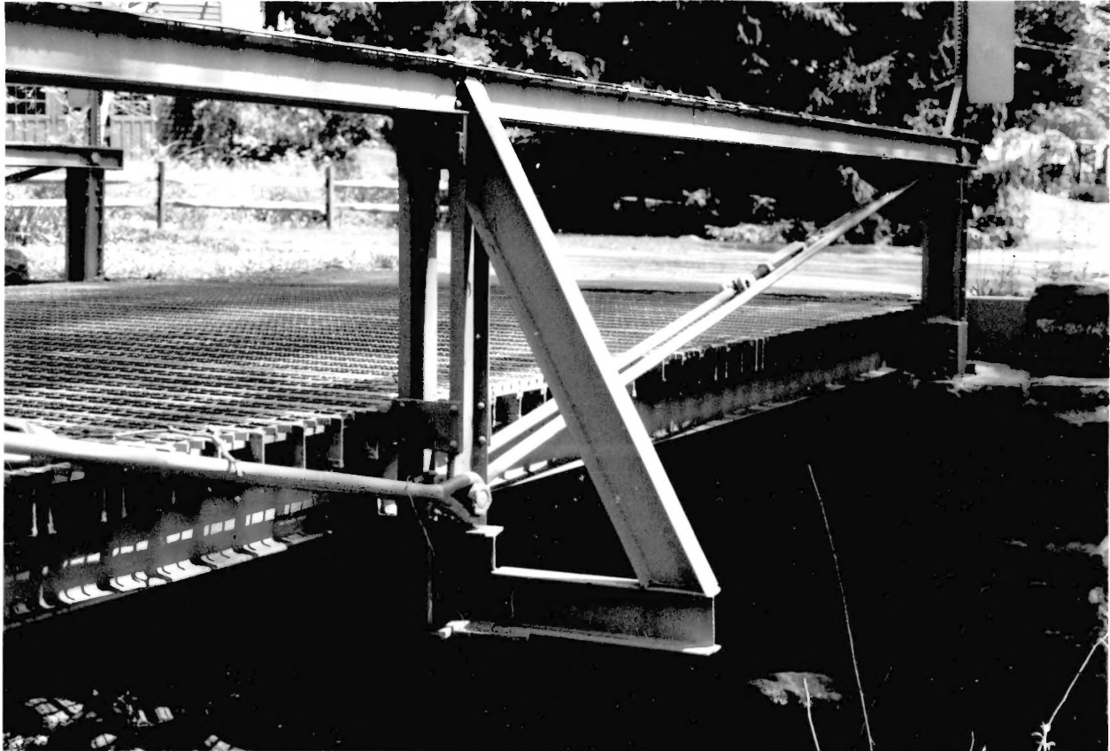
HOLLOW BROOK ROAD BRIDGE, TEWKSBURY TWP., HUNTERDON CO. PHOTO 50F5
