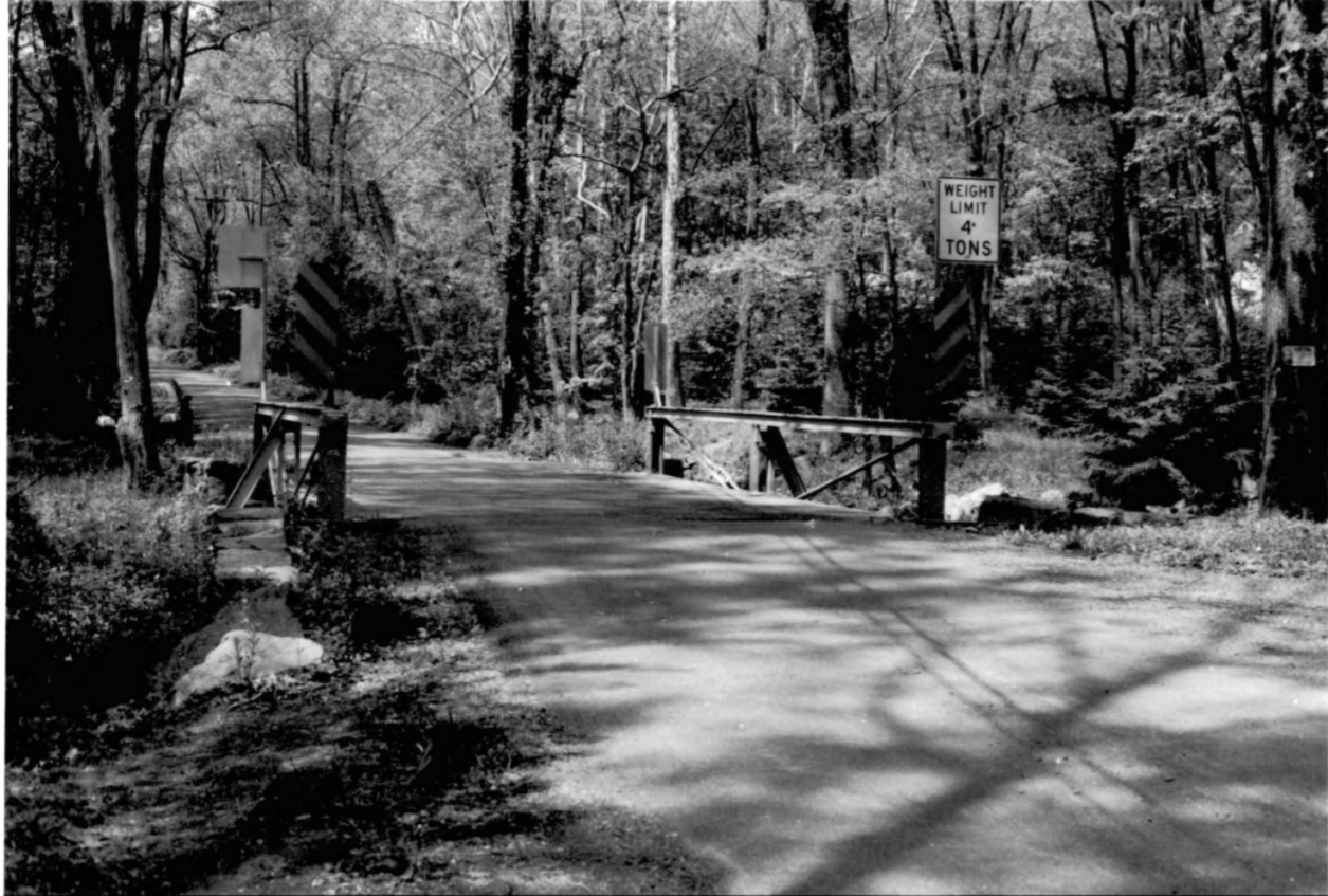
HOLLOW BROOK ROAD BRIDGE, TEWKSBURY TWP., HUNTERDON CO. PHOTO 2 of 5
