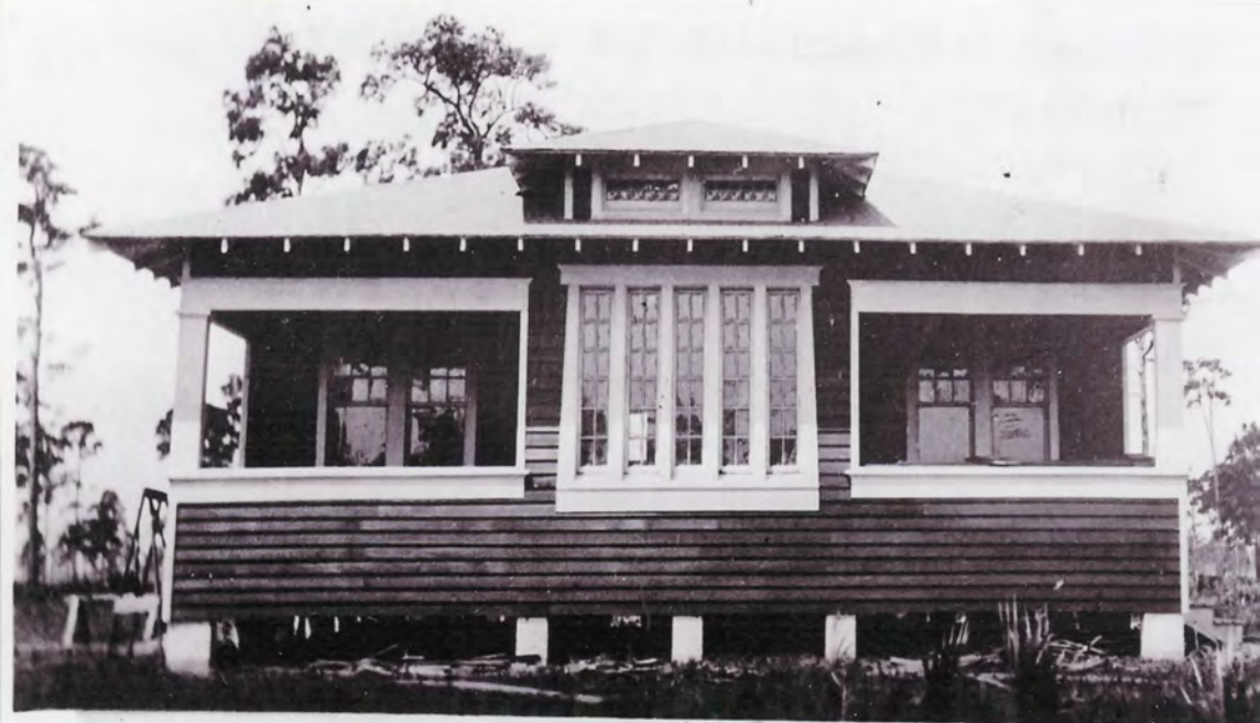
3 The first house in Osceola Park Addition to ero; the new home of Wm. H. Mills of Maitland,
