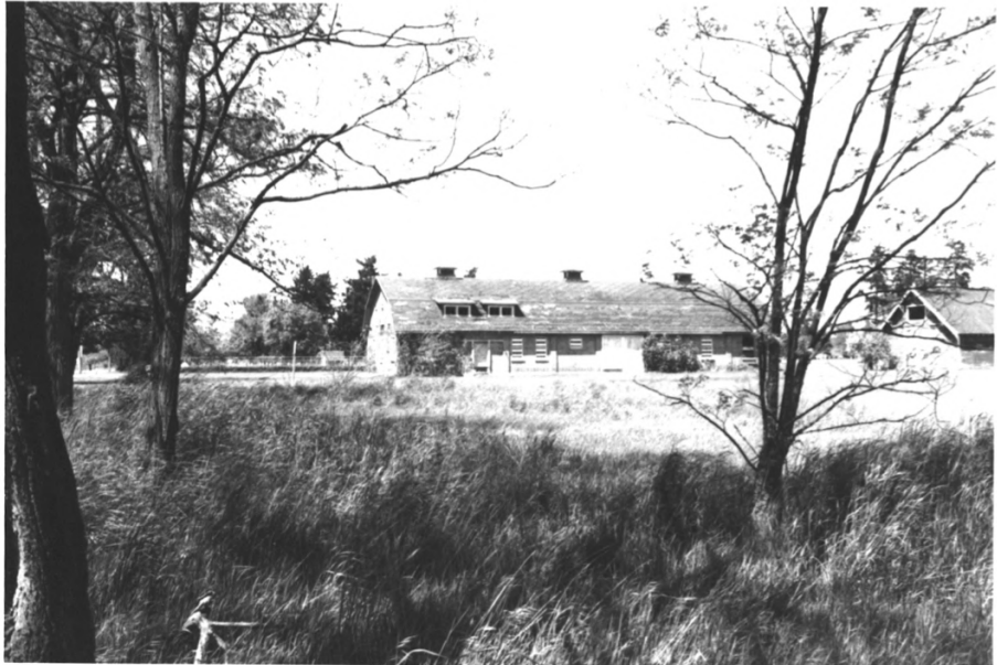
Fort Steilacoom District, Pierce Co, WA Photo 12 Addendum
