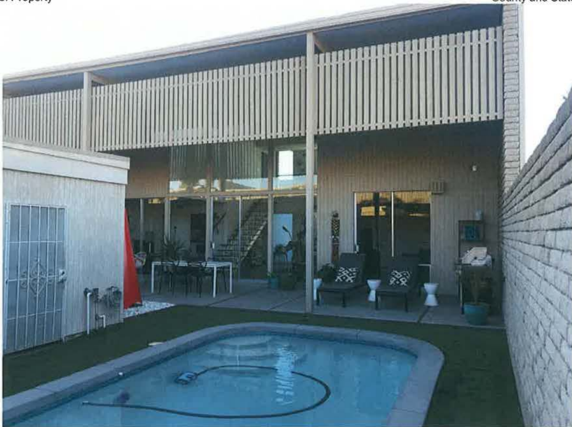
FIGURE #24: View of atrium – privacy screen, window wall, exposed post and beam
