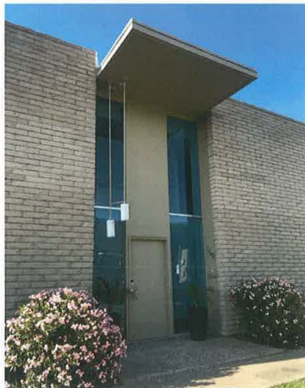
Figure #5: Building D - #1691 Entry with replacement glass
