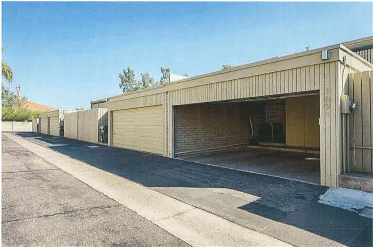
Figure #4: View of rear of Building D
