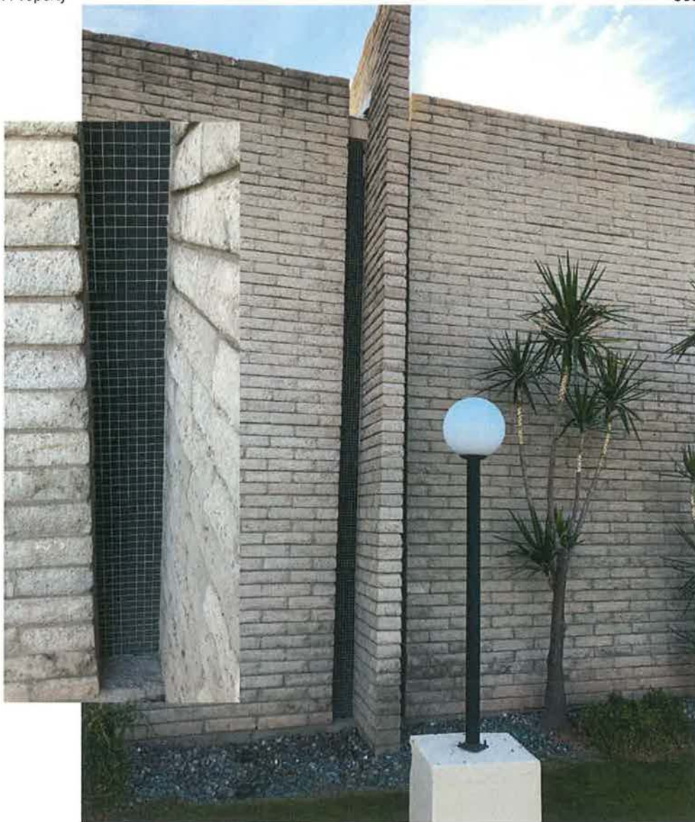
Figure #9: Building B – Mosaic tile detail
