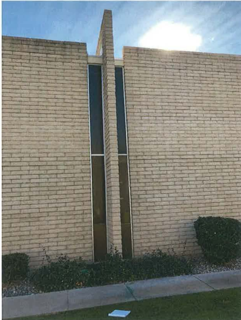
Figure #14: Building E kitchen window
