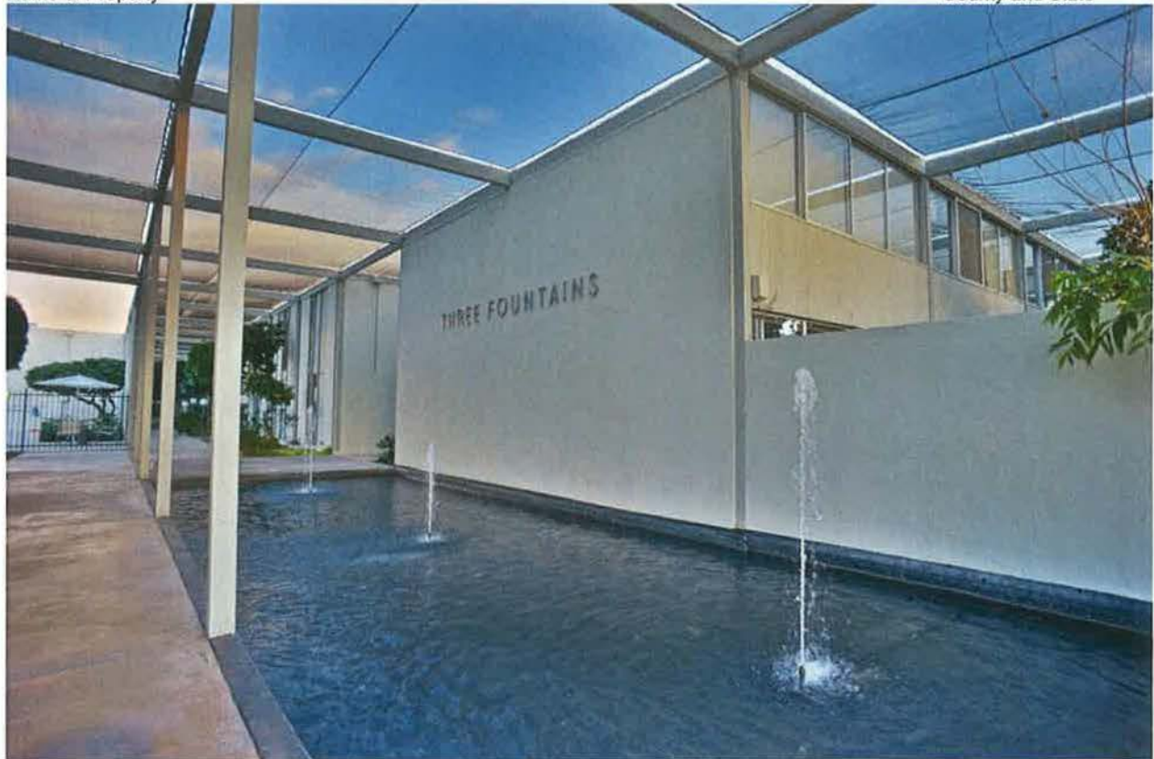
FIGURE #22: Three Fountains – Property entry and view of rear second floor windows https://azarchitecture.com/listing/three-fountains-al-beadle-architect-2/
