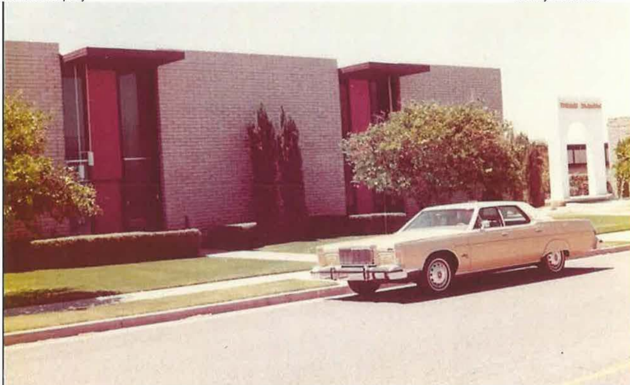
Figure #6: Building B – original paint scheme depicted at unit entries. Original fountain base.
