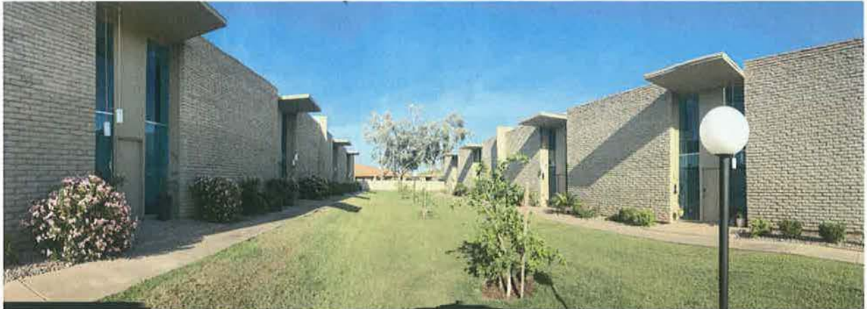
Figure #3: View facing east of Building D (left) and Building F (Right)
