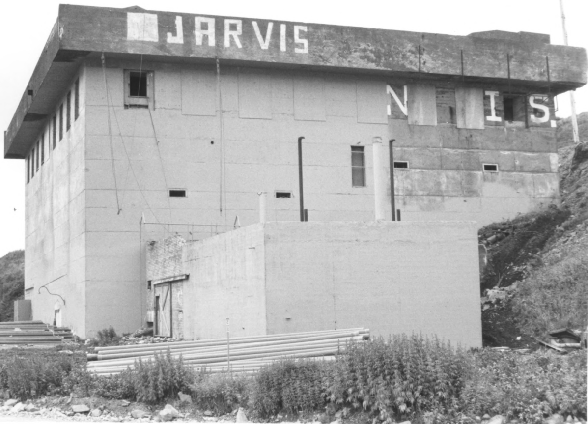
9. Navy's power plant at Dutch Harbor. Said to be strongest structure in the Aleutians, it can withstand a direct hit with a 500-pound bomb. It is presently being renovated to serve again as a power plant.
