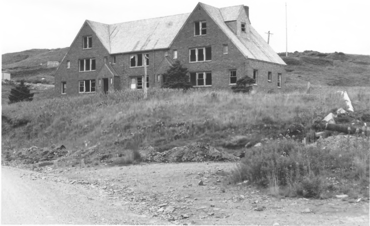
8. Pre-war naval residence at the naval radio station, Dutch Harbor. During World War II, chief petty officers occupied it, the only brick building in the Aleutians.
