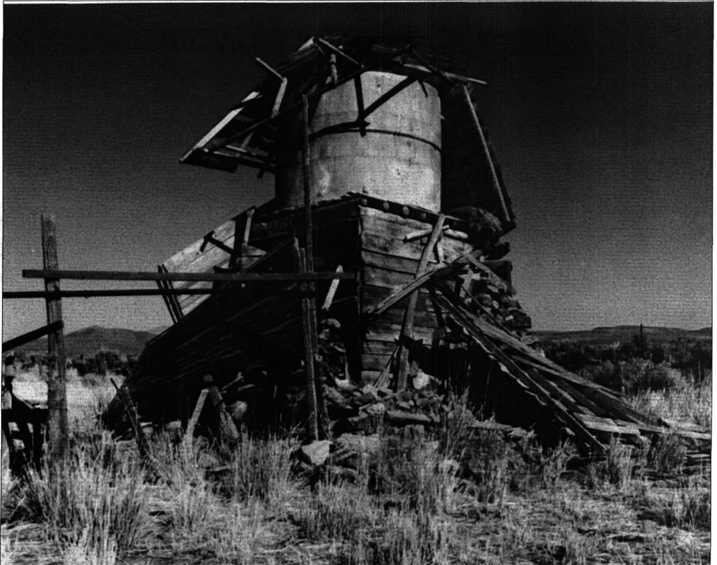
15 of 31: Exterior: Water tower, south and east facades, facing north, 2007
