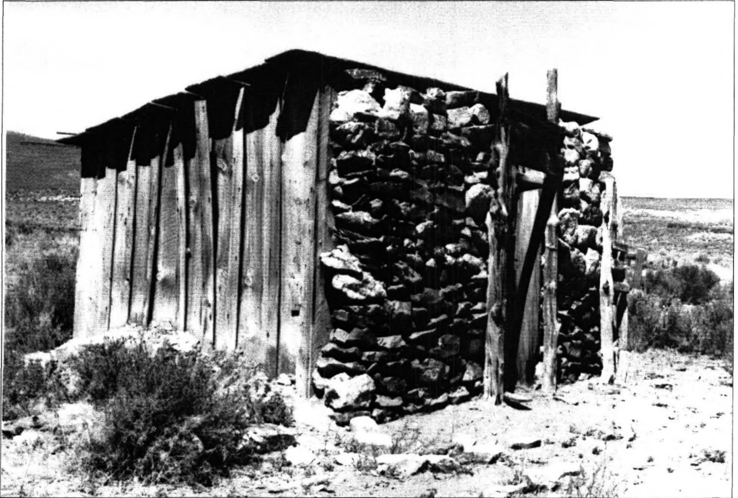
30 of 31: Reproduction: Rock shed, facing southeast, date unknown, Bureau of Land Management, Lakeview, Oregon
