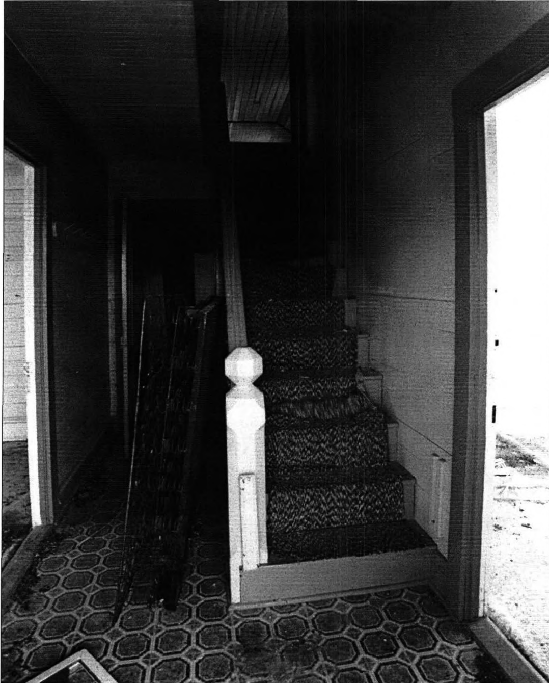
22 of 31: Interior Main Ranch House: Stairwell, facing north, 2004
