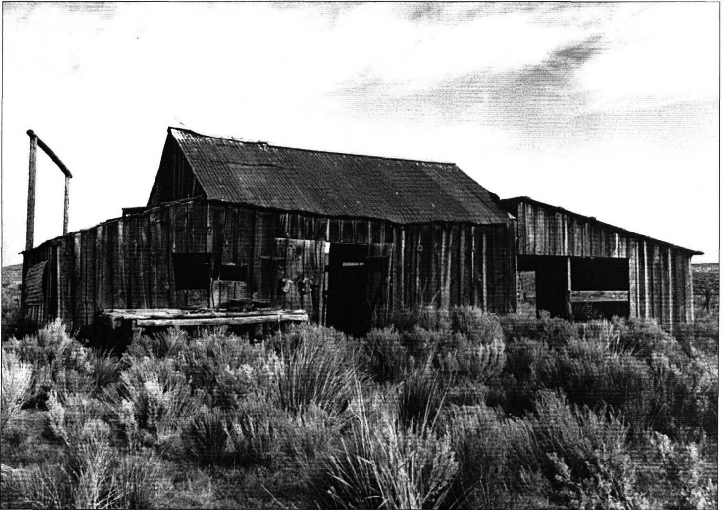
16 of 31: Exterior: Blacksmith shop, east façade, facing west, 2004
