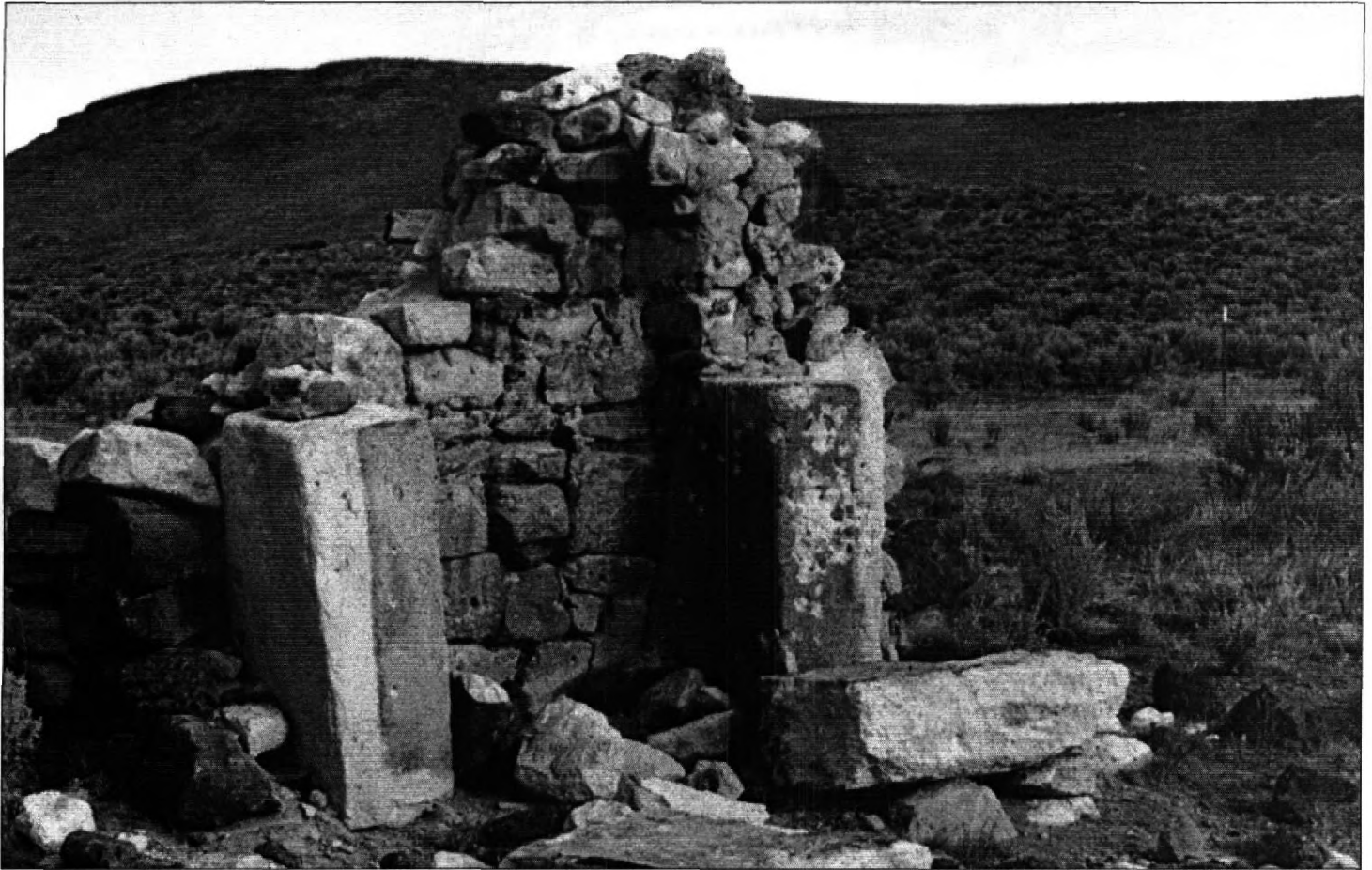
8 of 31: Exterior: Old ranch house fireplace (ruin), facing northwest, 2007
