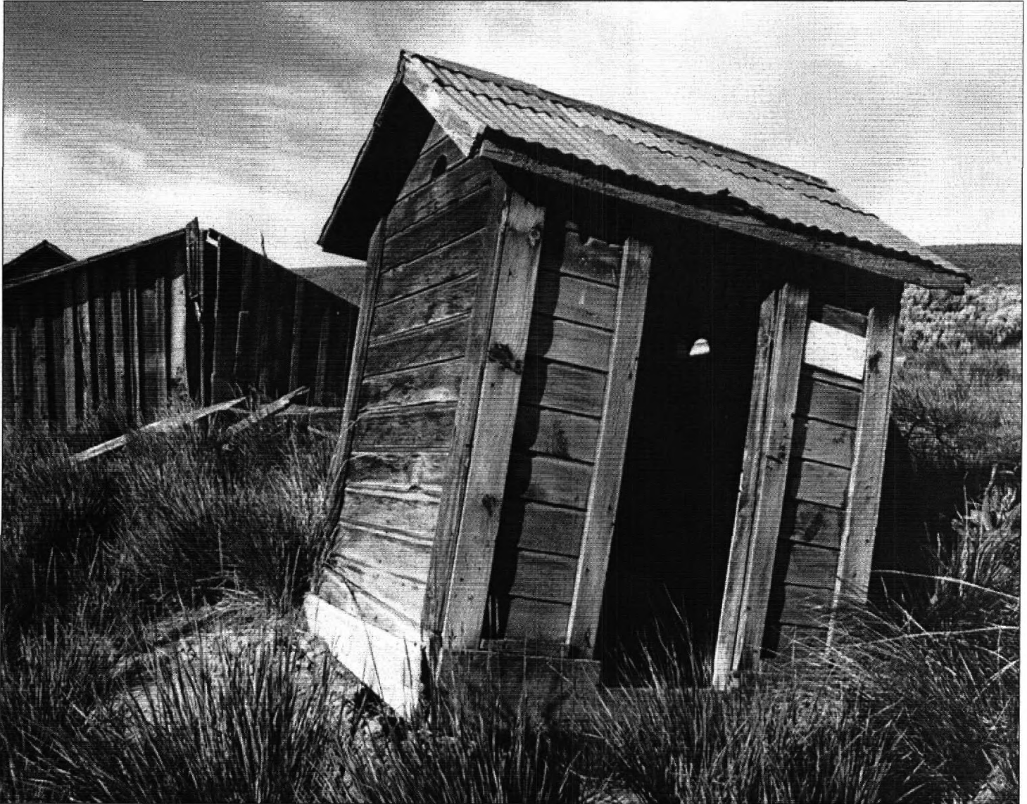
11 of 31: Exterior: Outhouse, south and east facades, facing northwest, 2004
