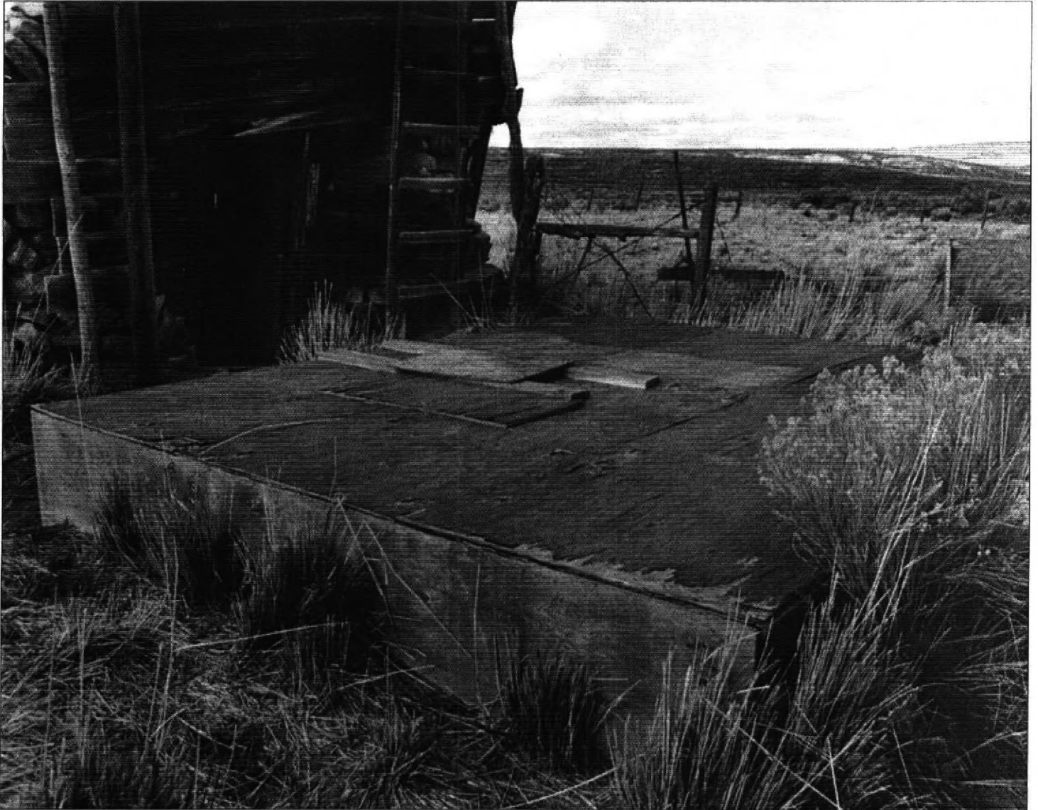
13 of 31: Exterior: Well, south and east sides, facing northwest, 2004
