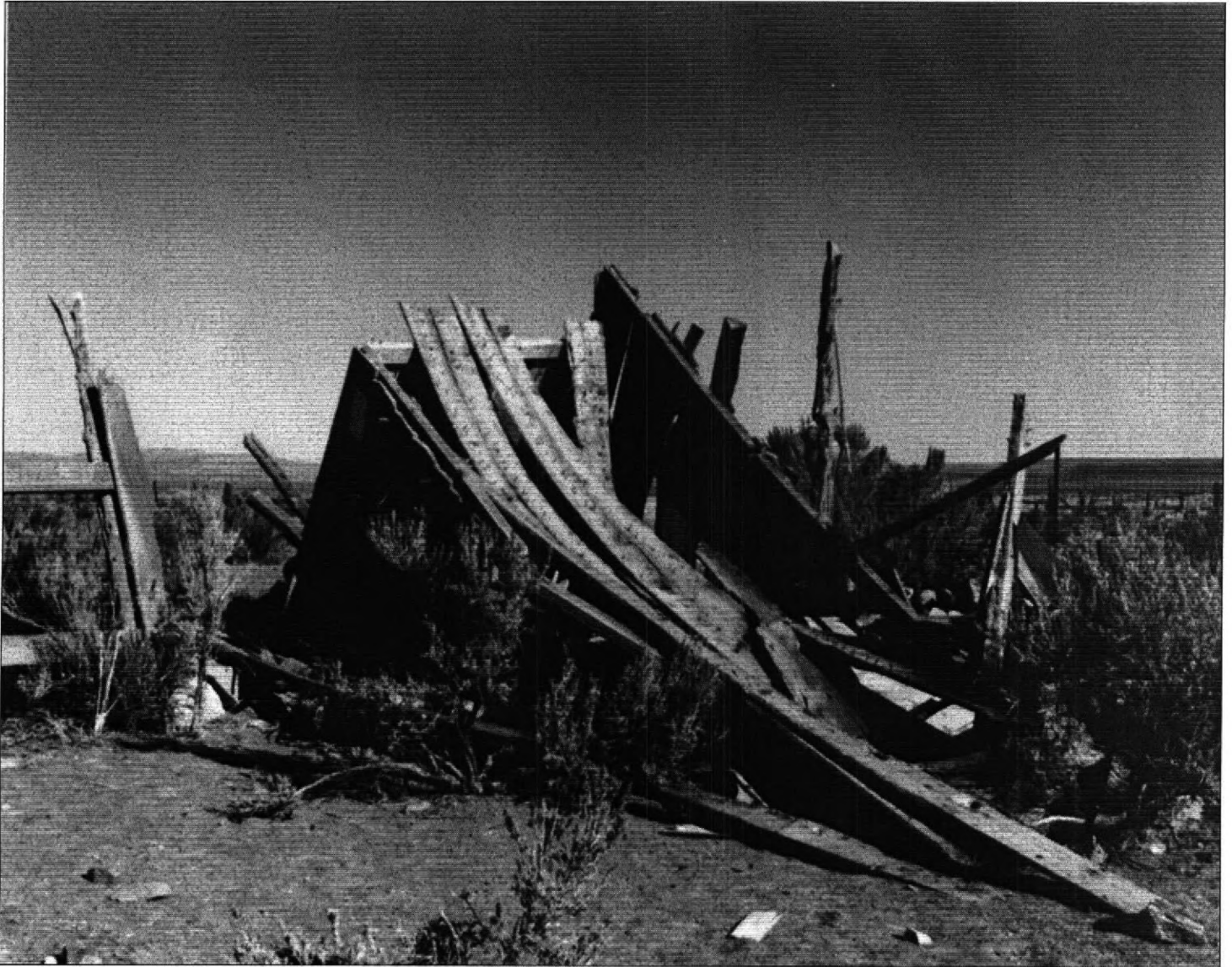
18 of 31: Exterior: Rocked shed, south façade, facing northeast, 2007
