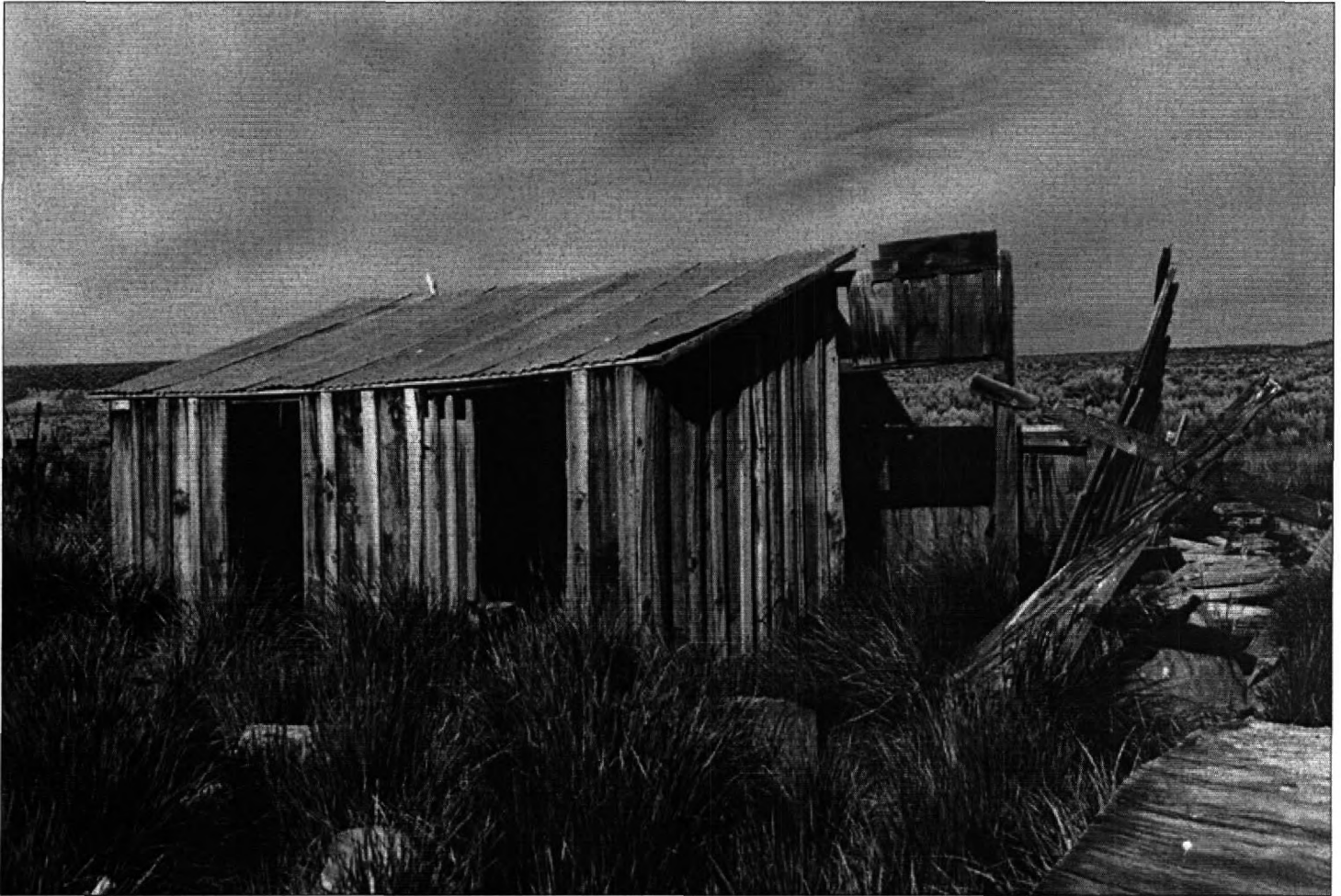
10 of 31: Exterior: Woodshed, north and east facades, facing southwest, 2004
