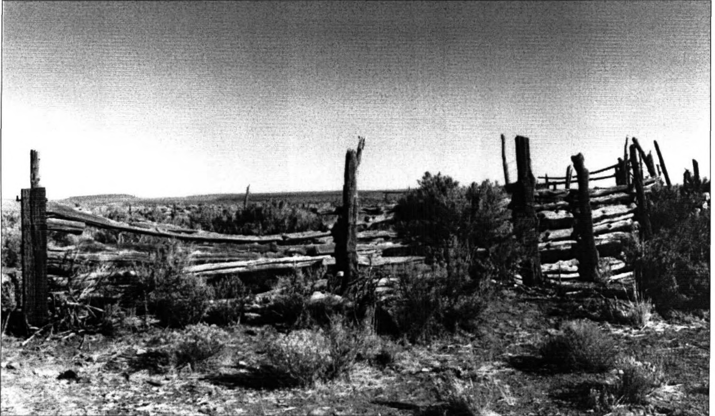
17 of 31: Exterior: Fencing, facing east, 2007
