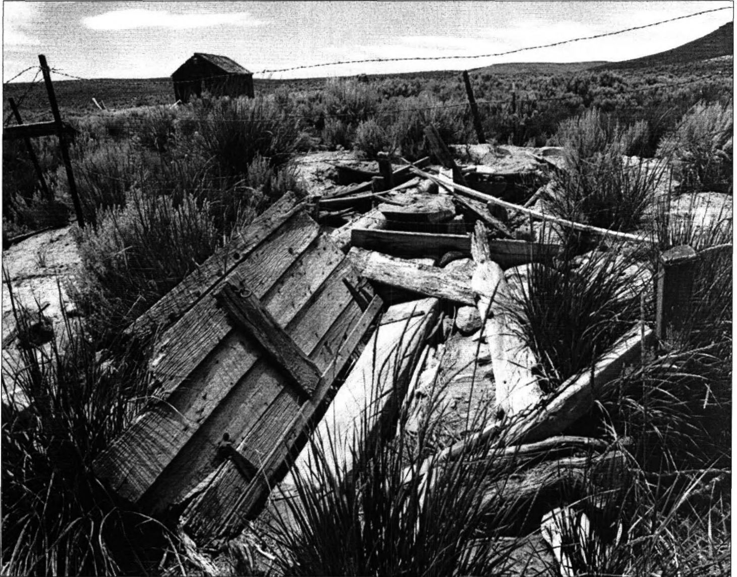
9 of 31: Exterior: Root cellar, east side, facing west, 2004
