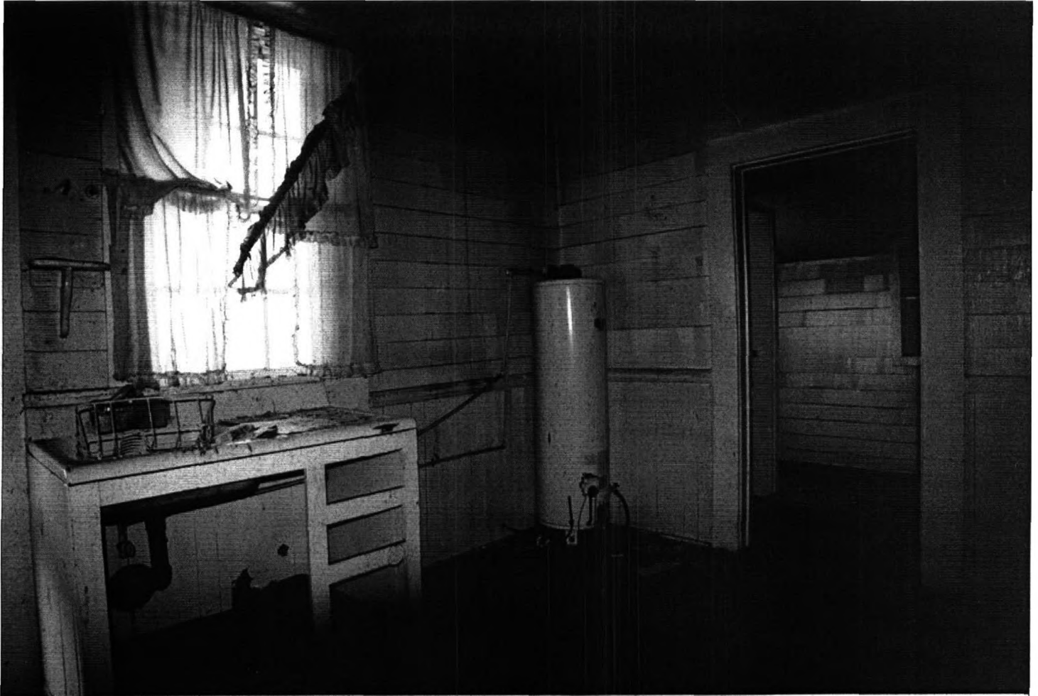
26 of 31: Interior Main Ranch House: Kitchen/shower, facing northeast, 2004
