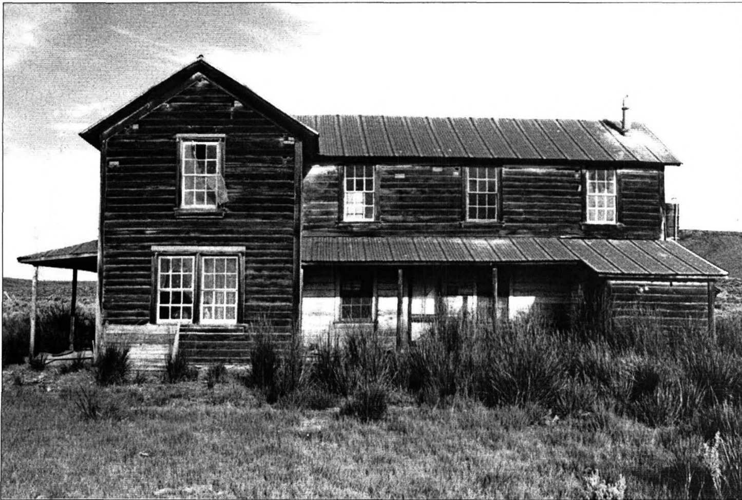
4 of 31: Exterior: Ranch house, east façade, facing west, 2004
