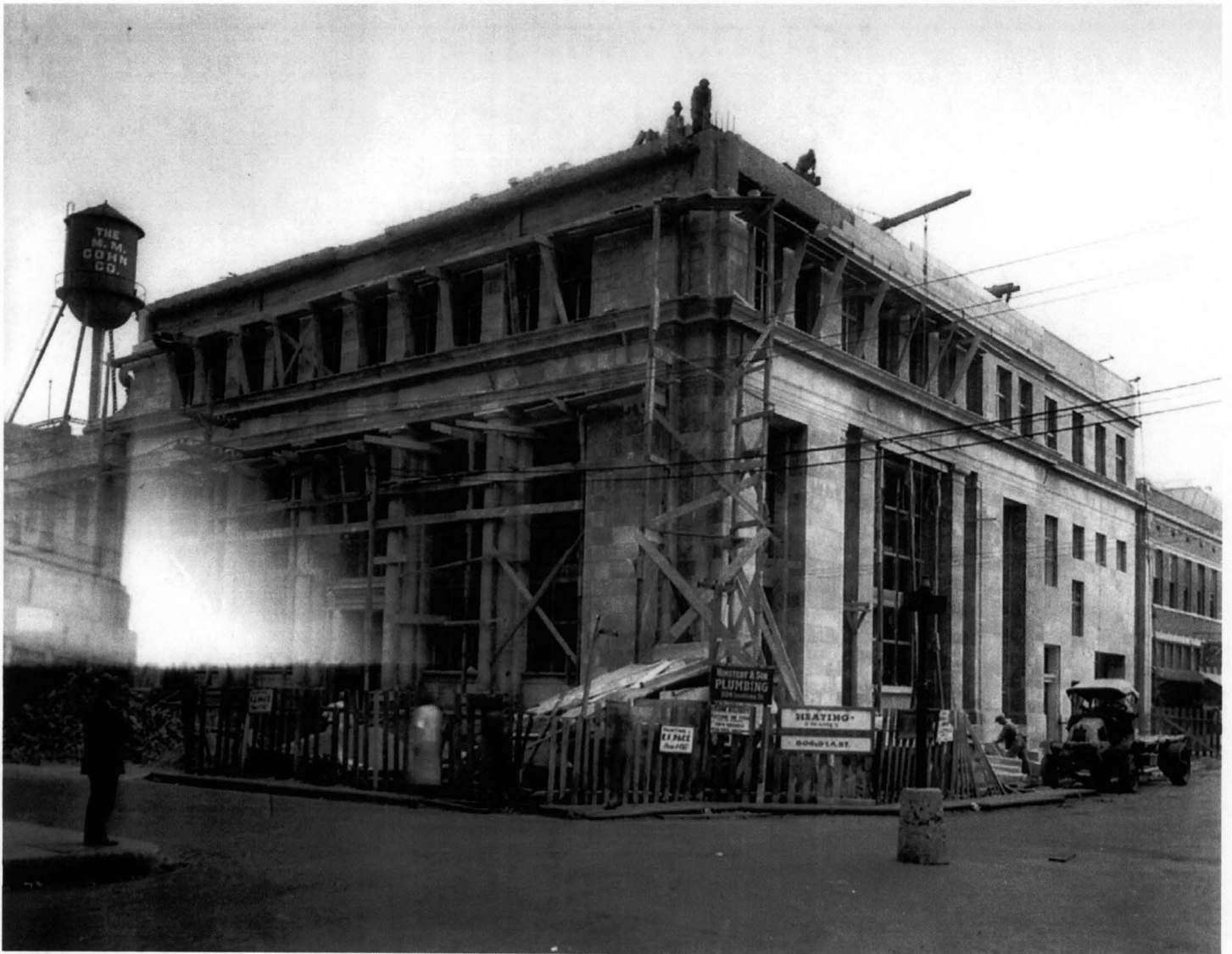
Figure 9: Federal Reserve Bank Building under construction, 1924 (From the files of the Arkansas Historic Preservation Program)
