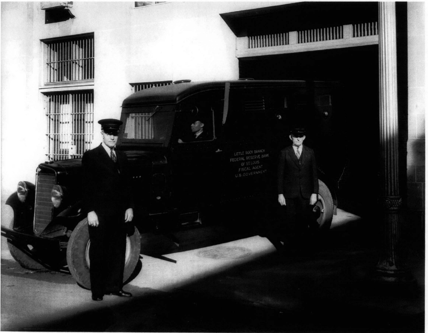
Figure 10: Armored truck at the Federal Reserve Bank Building, c.1925 (From the files of the Arkansas Historic Preservation Program)
