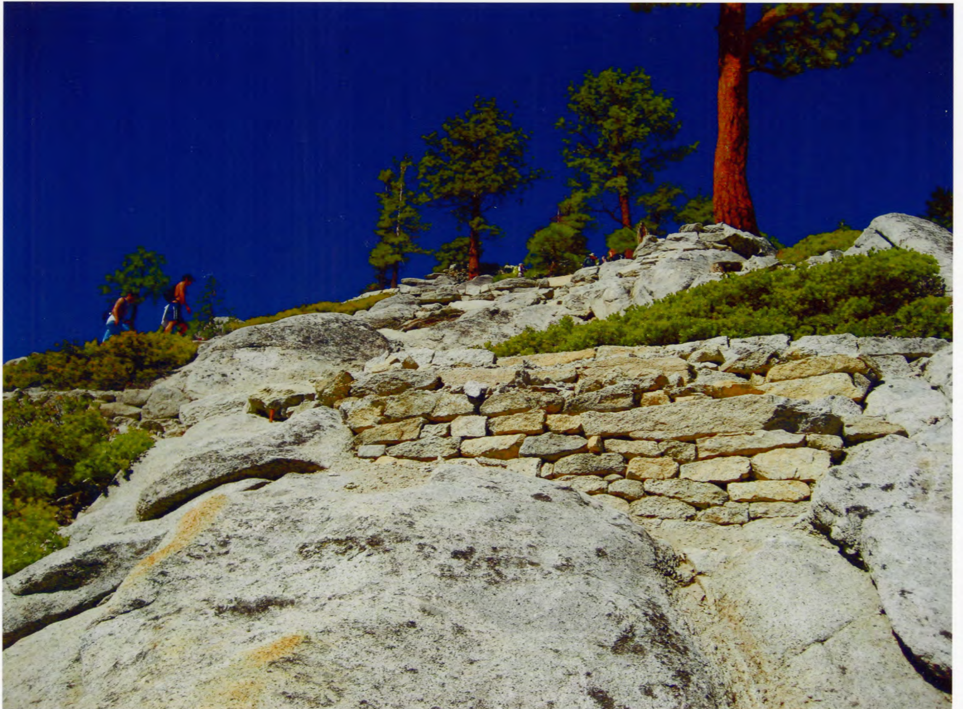
CA_Mariposa County_Half Dome Cables and Trail_0004
