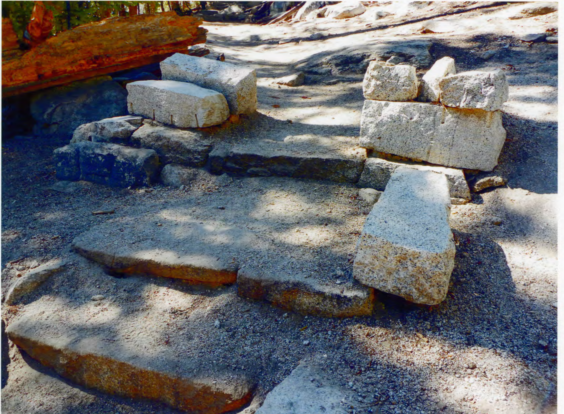
CA_Mariposa County_Half Dome Cables and Trail_0001
