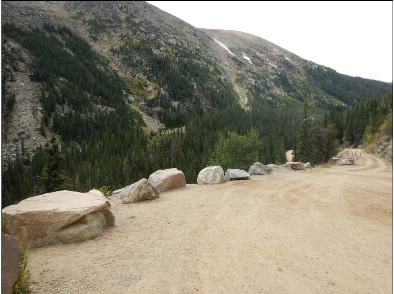
Photograph 4. Boulder curbing, camera facing southwest. CO_LarimerCounty_Fall River Road_Amendment_Boundary Increase_Rocky Mountain National Park MRA_0004
