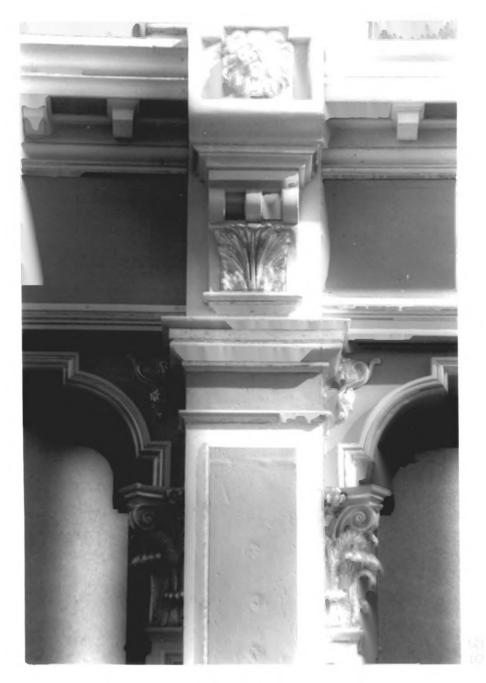
ZCMI Cast Iron Front 15 South Main Street, SLC, Ut. October, 1976 NOV 5 1976 Taken by Harold Carpenter detail at intersection of mullion bilaster and beam South Like City, with
