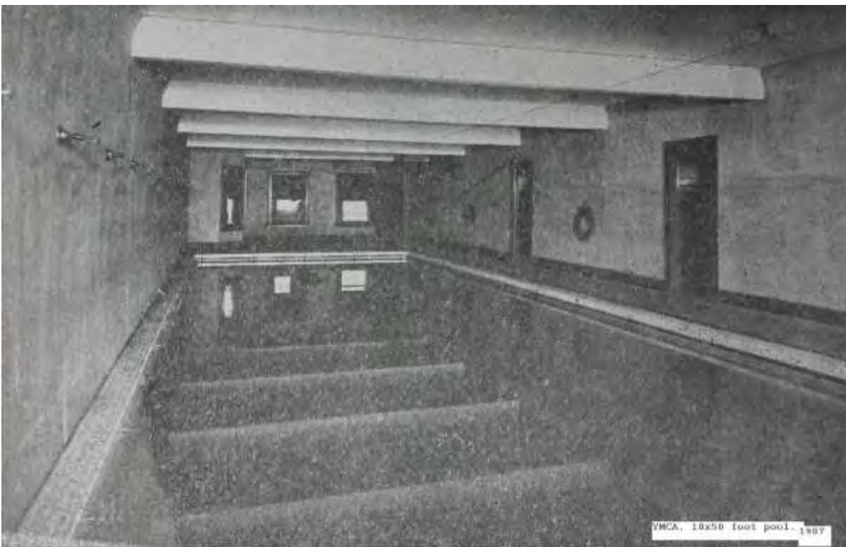
Fig. 21. Walla Walla, WA YMCA. Natatorium (indoor swimming pool), at daylight basement west, view looking north, 1907. Source: Penrose Memorial Library collections, Whitman College.
