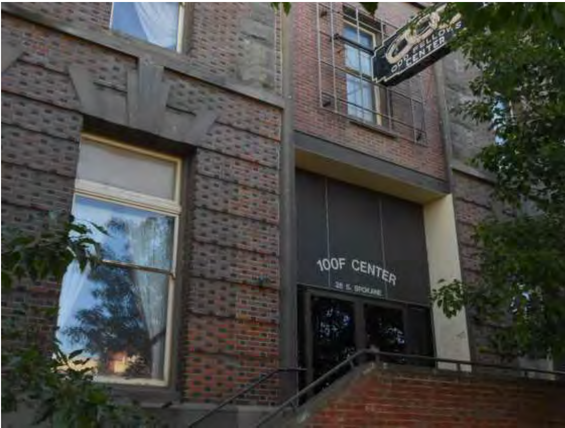
Fig. 4. Walla Walla, WA YMCA. Entry at 28 S. Spokane St., including 1907 masonry with 1948 alterations to entry bay, looking NW, June 2014. Source: Stephen Day Architecture.
