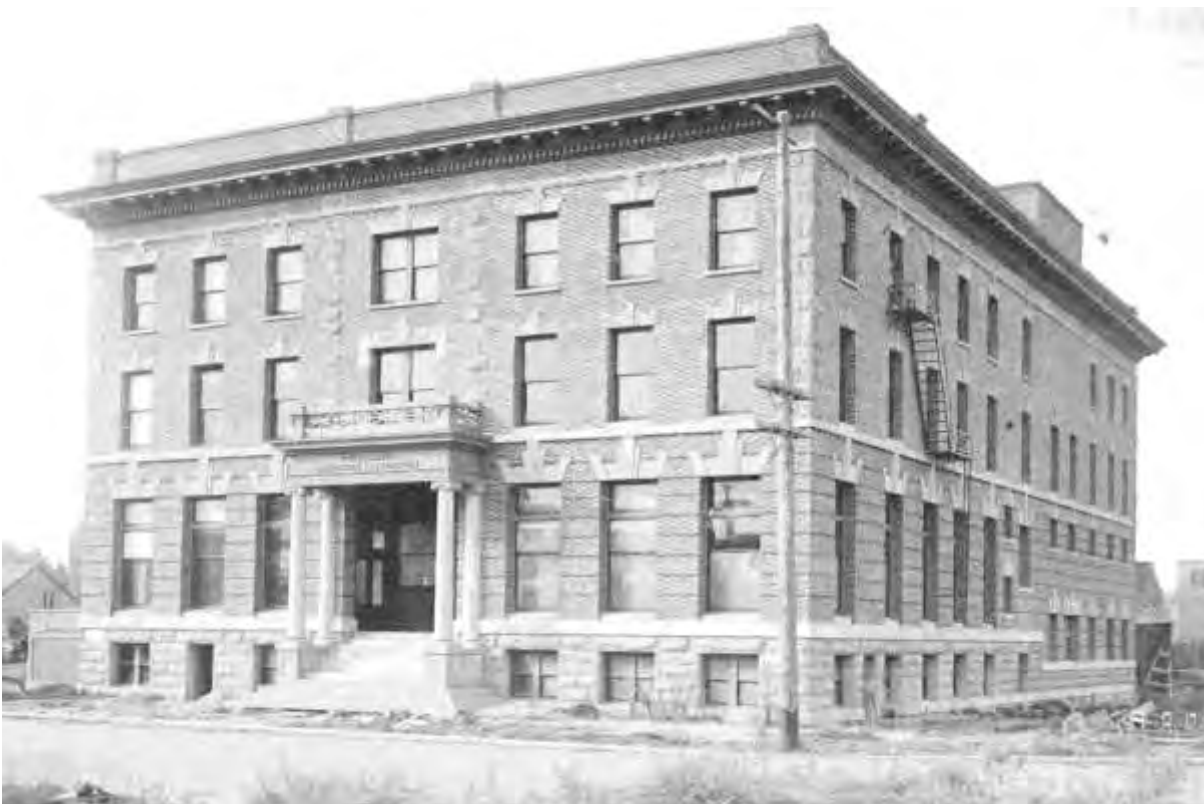
Fig. 2. Walla Walla, WA YMCA. Building nearing completion of construction, looking southwest, 1907. Source: Penrose Memorial Library collections, Whitman College.
