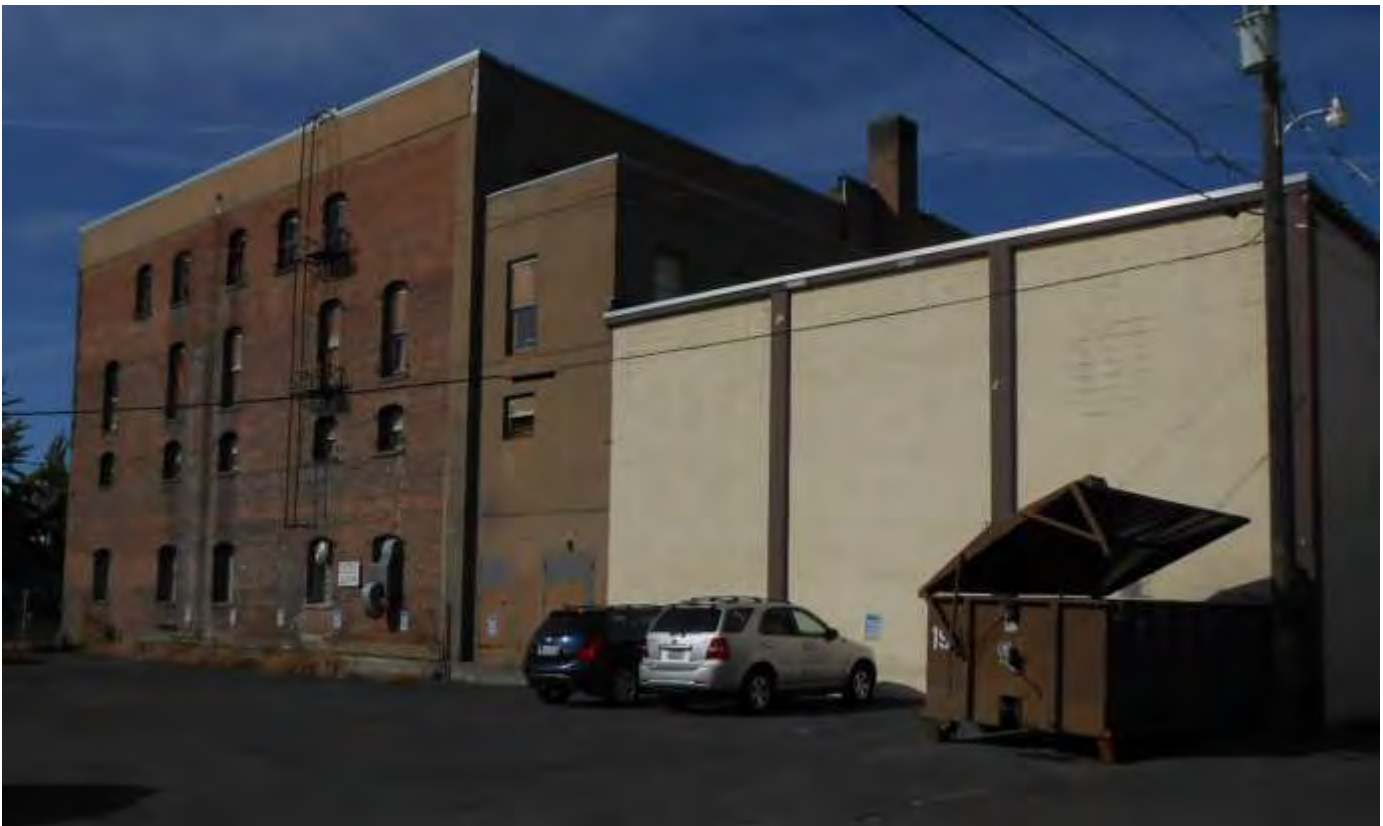
Fig. 13. Walla Walla, WA YMCA. West elevation, with (L to R): 1907 building, noncompatible 1948 and 1959 additions, looking NW, June 2014. Source: Stephen Day Architecture.
