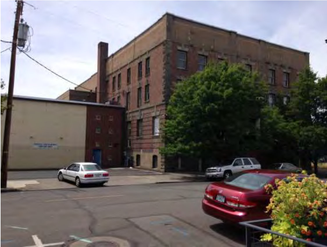
Fig. 3A. Walla Walla, WA YMCA. 1907 building with noncompatible 1959 addition on left, view looking NW from S. Spokane Street, June 2014. Source: Stephen Day Architecture.
