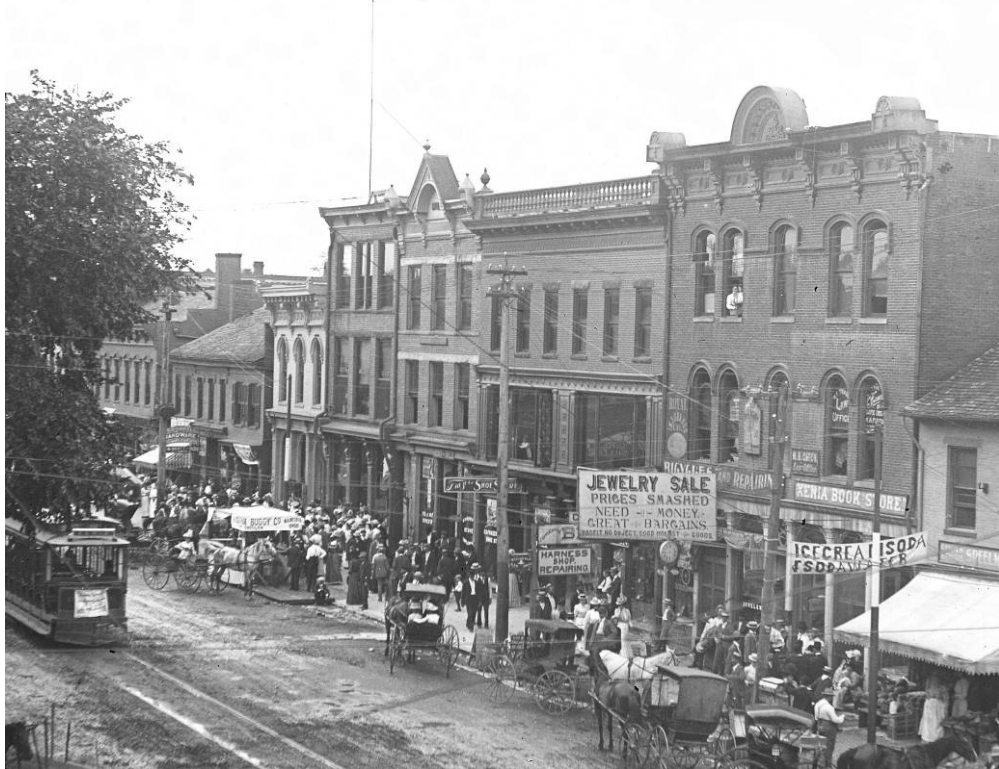
Image 13. View of south side of E. Main Street, looking southeast, 1894.
