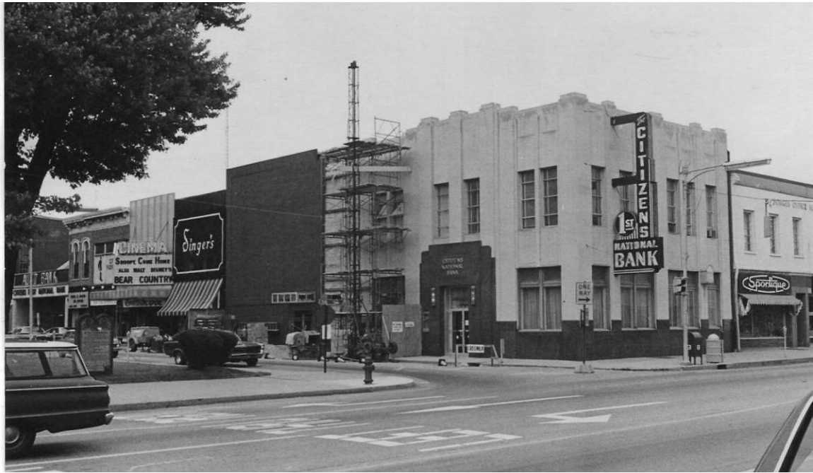
Image 23. View of Greene Street, looking northeast, 1972.
