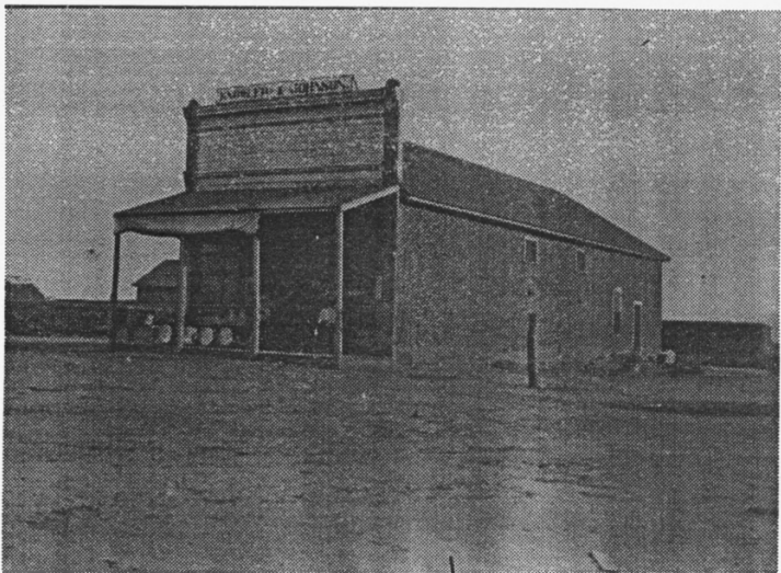
Historic Photo of the Knowler & Johnson Store (now Bonita Store), c. 1885 showing the brick-pattereded tarpaper siding.
