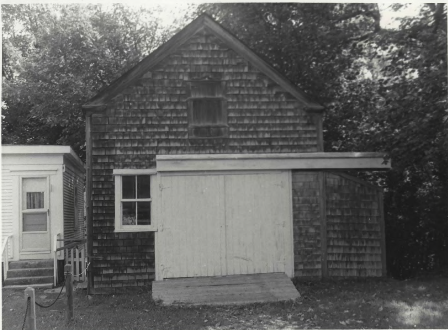
Barn facing Holbrook Avenue but part of Main Street property 67 - Sheet 120 - 22 Photo 19
