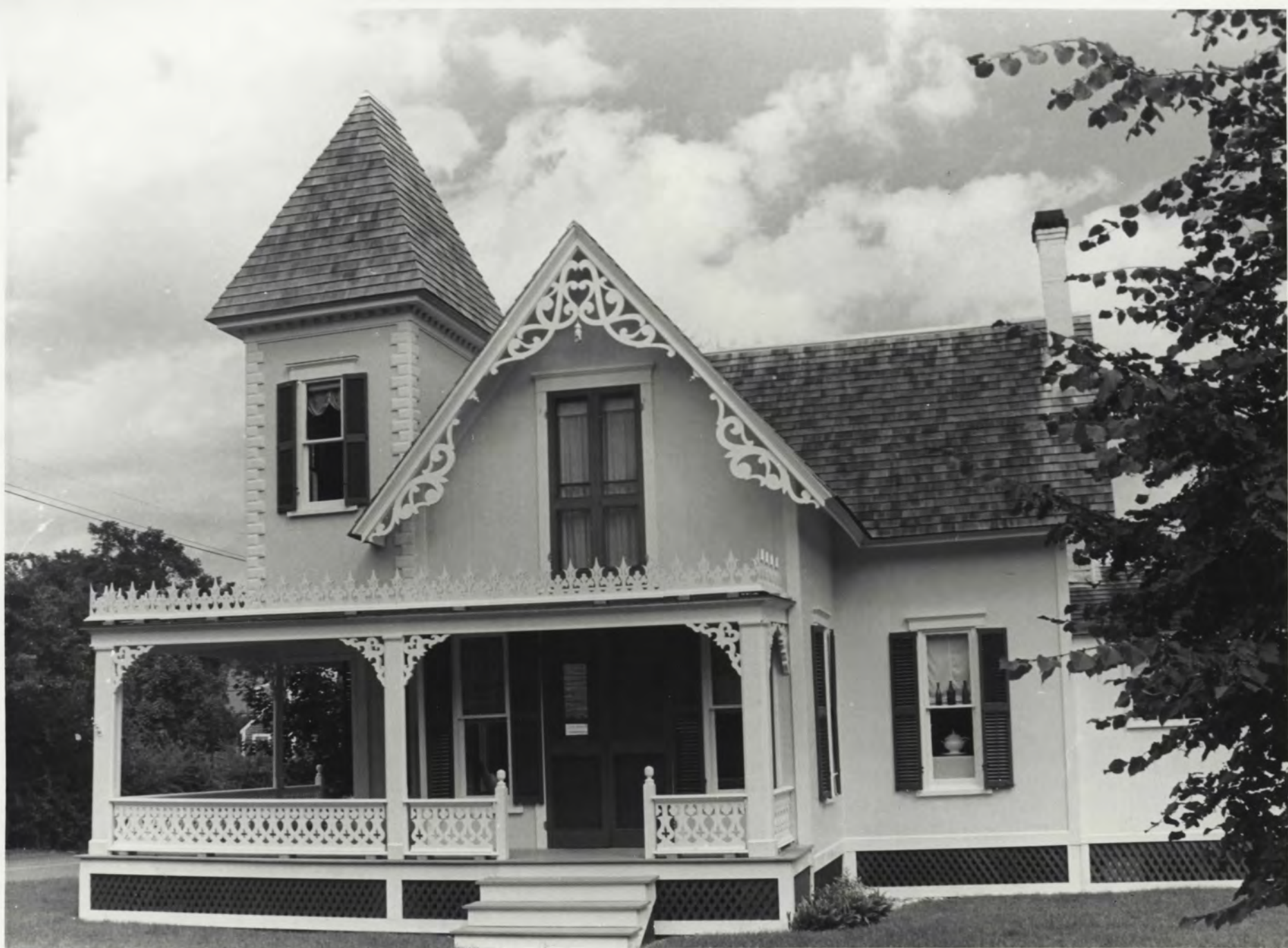
Carpenter Gothic, Halbrook Avenue Wellfleet 84-Sheet 120-22 Photo 18
