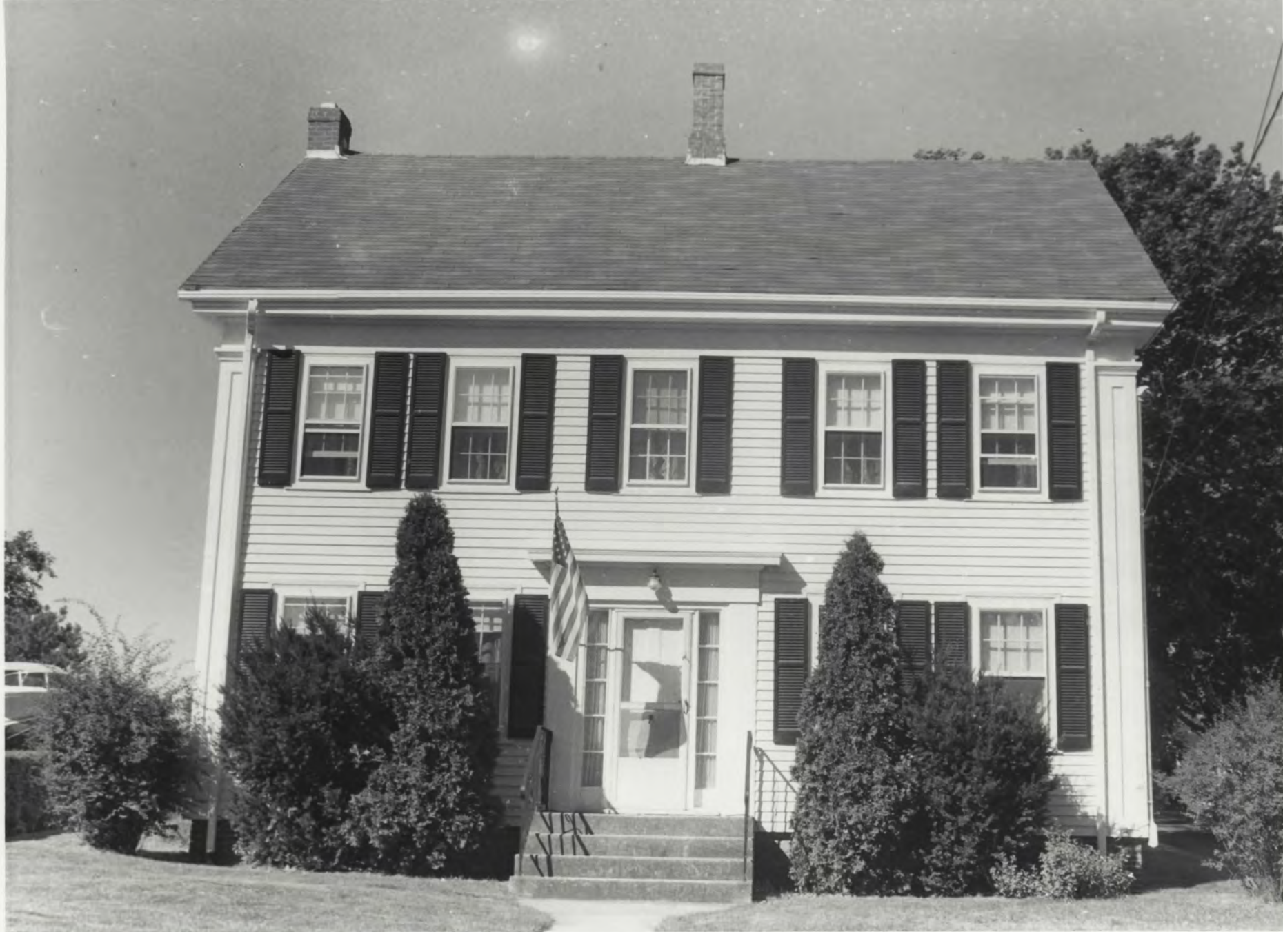
Transitional Federal style house, c1820 Commercial Street, Wellfleet # 20 - sheet 123-22 Photo # 11
