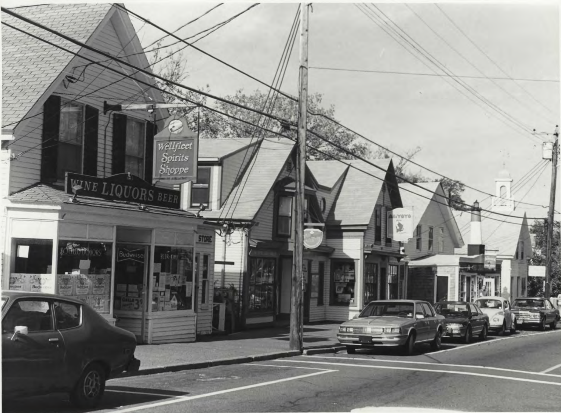
Wellfleet's Greek Revival Photo #1 Main Street (72-75A - sheet 120722)
