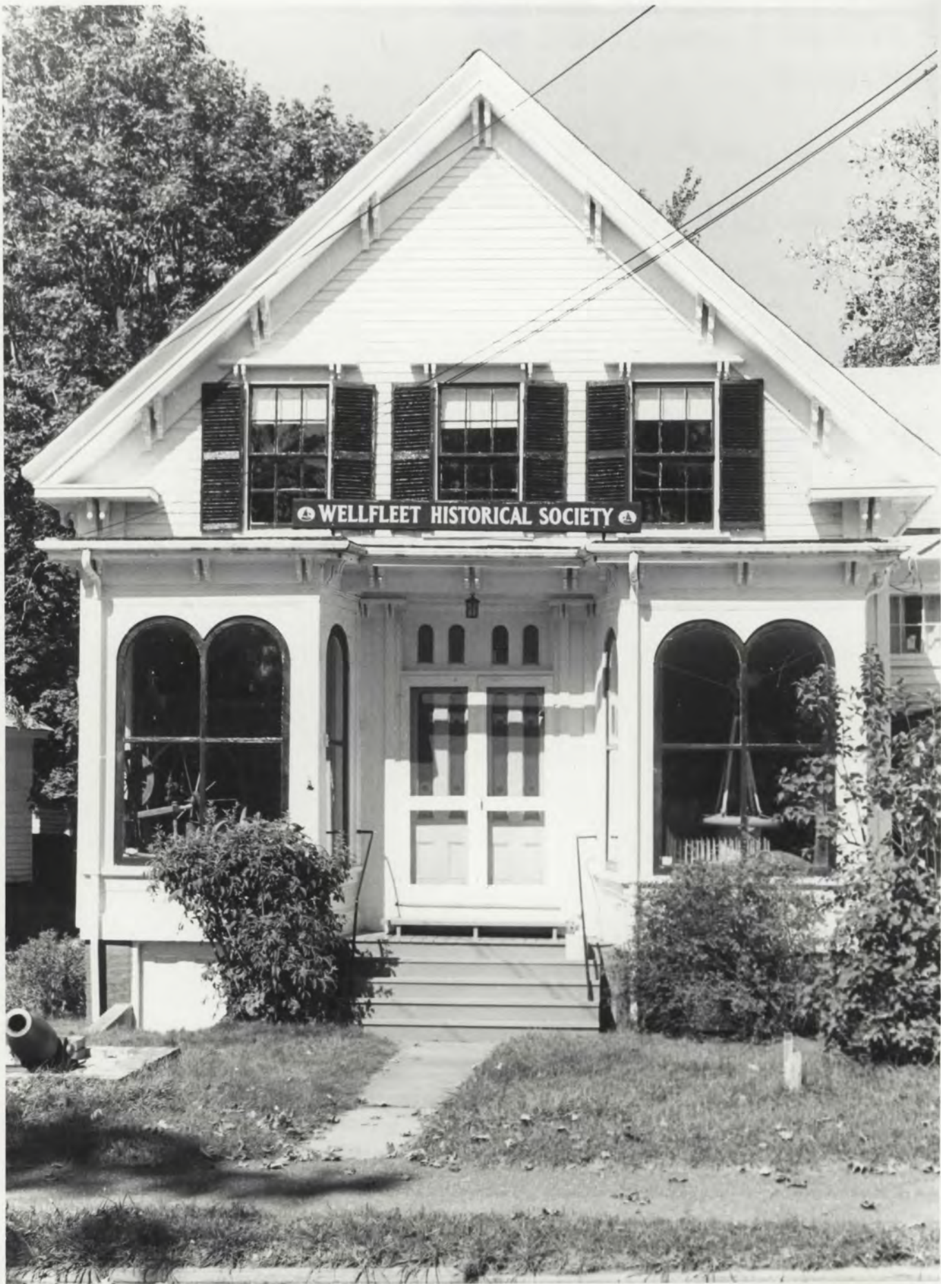
Park of multi-owner buildings Main St., Wellfleet 5 Sheet 121-22 Photo 15
