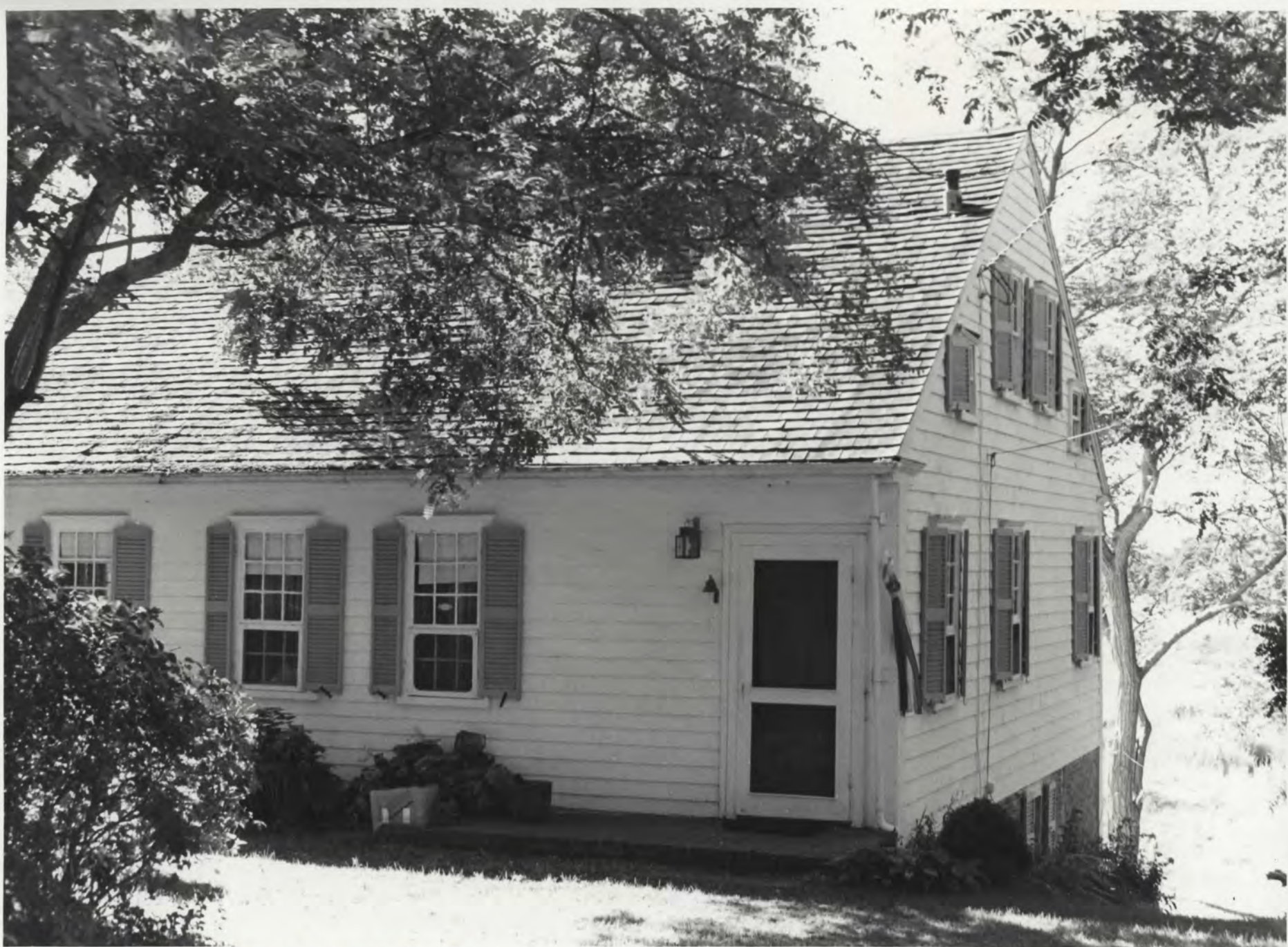
3/4 Cape moved from Griffith's Island to site off East Commercial Street - Rear side view Photo 4 (64 - sheet 121-22) Wellfleet
