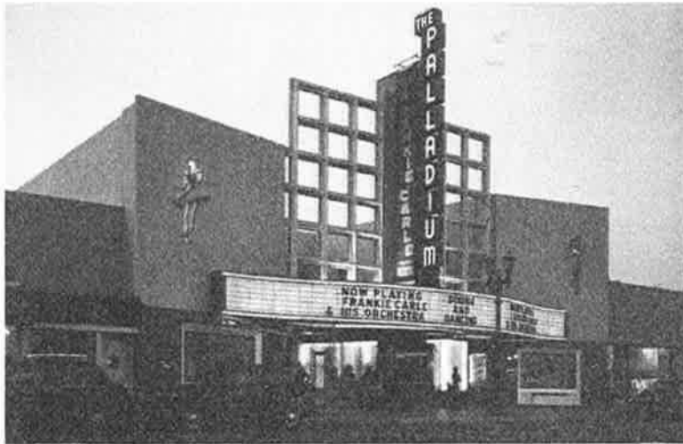
Figure 16. Primary façade, view looking northeast, n.d. Source: Hollywood Heritage
