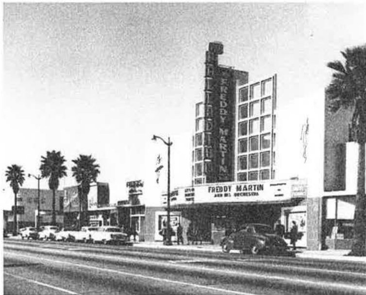
Figure 12. Primary façade, view facing northwest, 1949. Source: Bison Archives (Marc Wanamaker)
