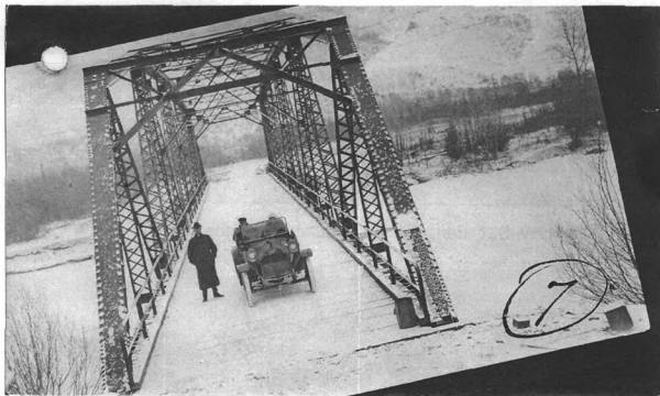
Photograph 0002. West portal. Browne's Bridge. View to the east.
