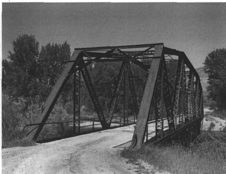
Photograph 0001. East portal and north profile. Browne's Bridge. View to the west.
