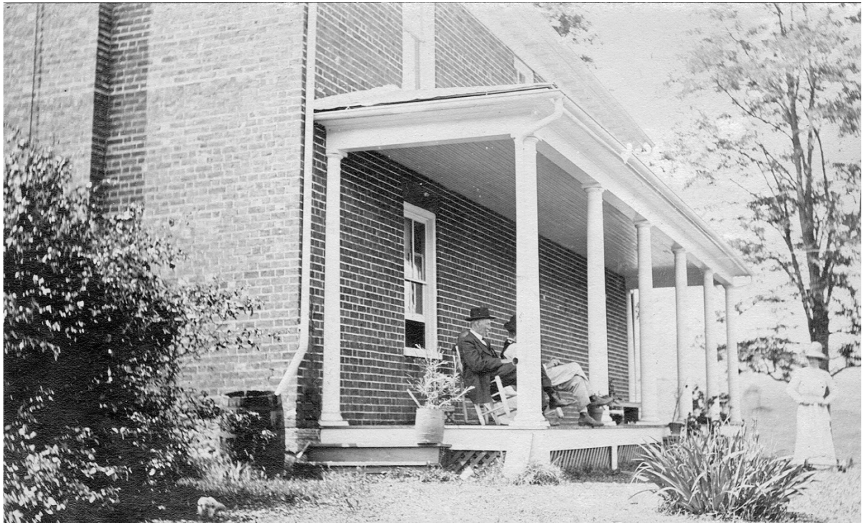
Figure 4. The wooden-columned front porch, circa 1910.
