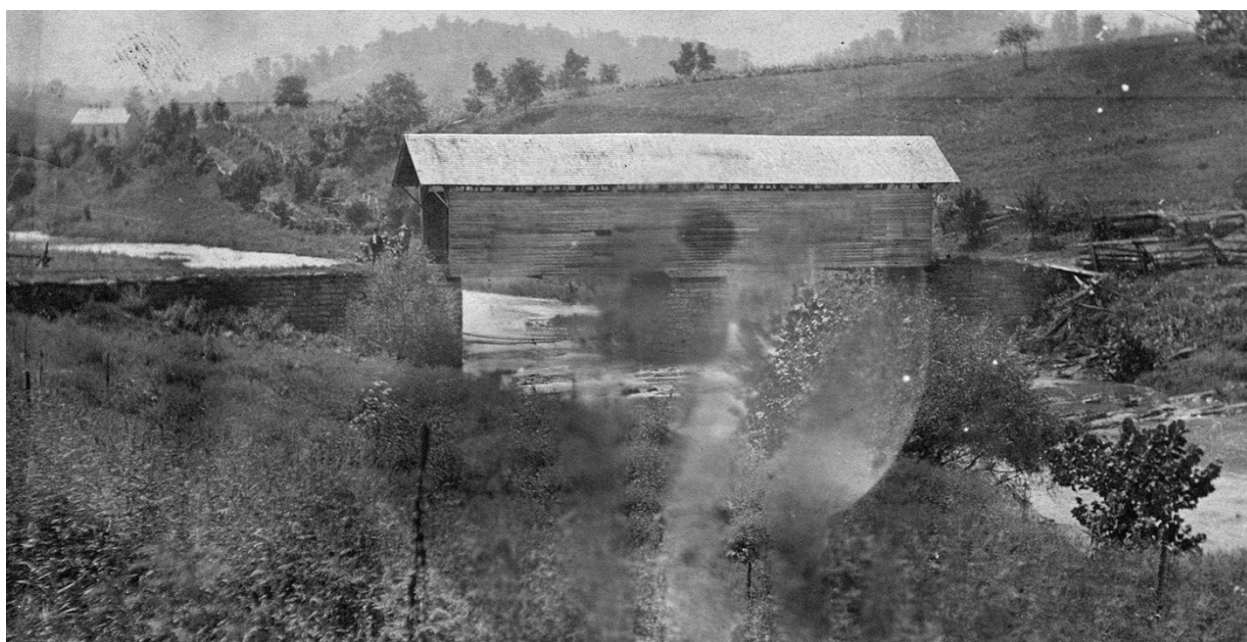
Figure 1. The covered bridge spanning Big Cedar Creek, facing south, circa 1900.
