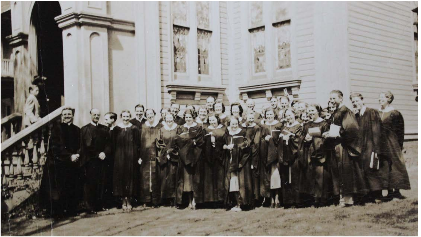
First Reformed Church, south façade and entrance, undated historic photograph
