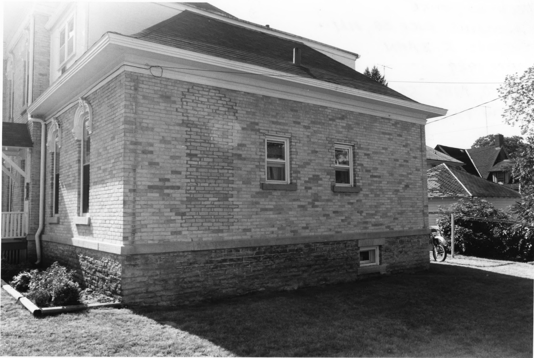
HOLMAN HOUSE FARIBAULT RICE CO., MN PHOTO I.D. 09930 #1
